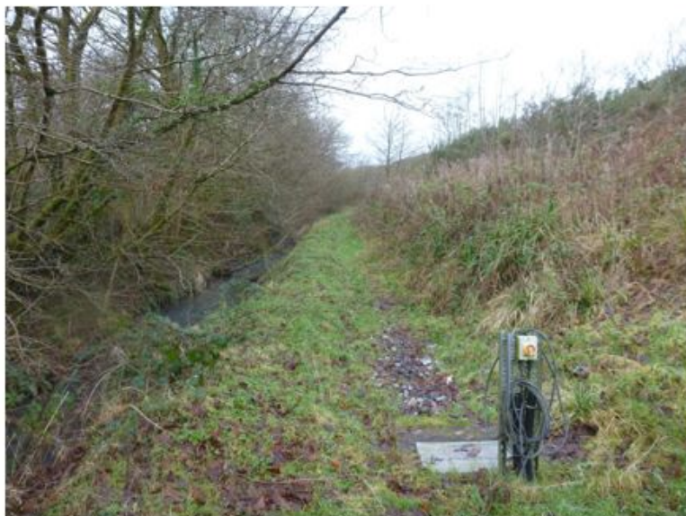
Photograph showing French drain and heavy vegetation along landfill flank. No visual evidence of breakouts were noted.
