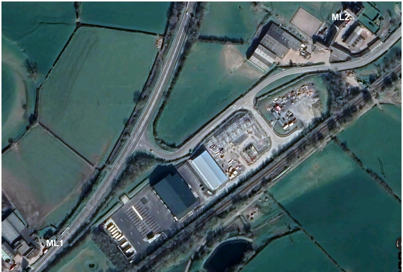
Figure 5-1 – Aerial view of the off-site monitoring locations
