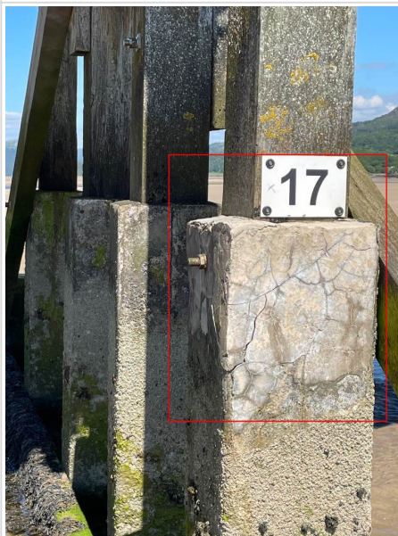
Repairs at span 17
