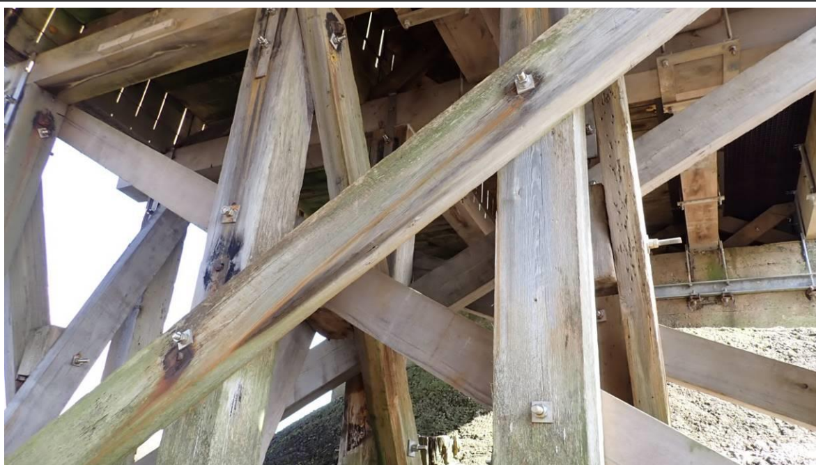
Photo 5 All steel fixing, have been replaced
