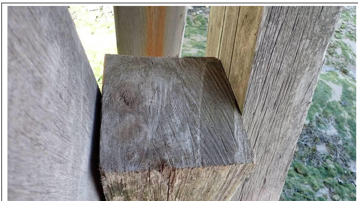
Photo 4 New wedge between piles 4 and 5
