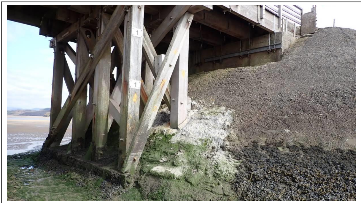
Photo 1 Low Mileage abutment and Trestle 1
