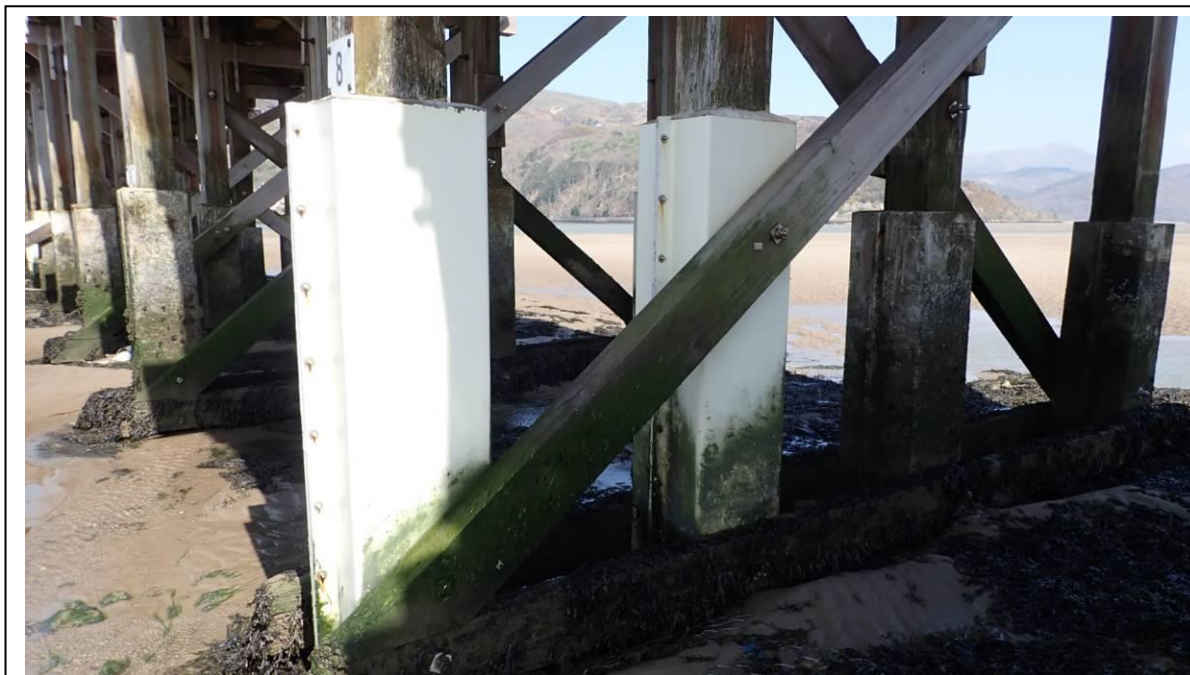
Photo 13 Trestle 8 – Pile 1, new encasement
