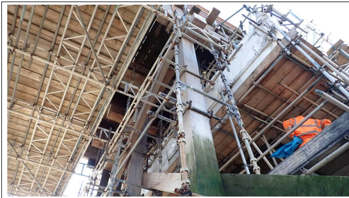
Photo 37 Trestle 112 – Pile 4, new encasement
