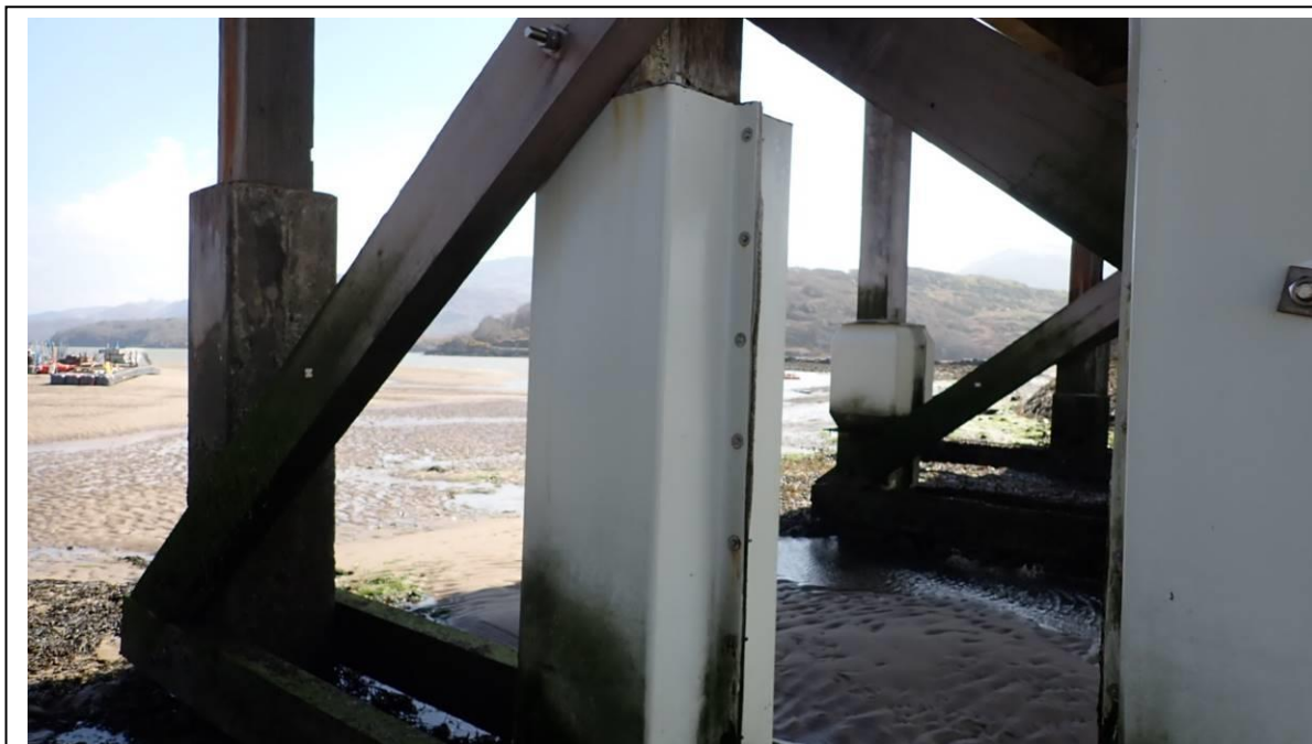
Photo 11 Trestle 4 – Pile 3, new encasement
