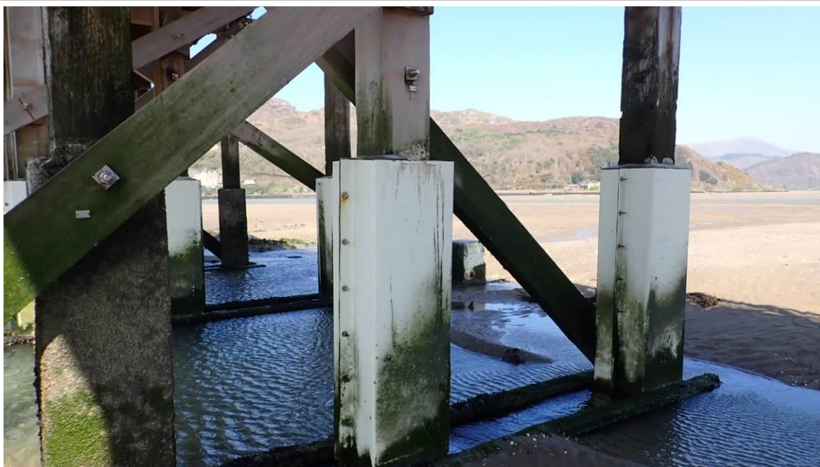
Photo 21 Trestle 21 – Pile 2 – Encasement in fair condition
