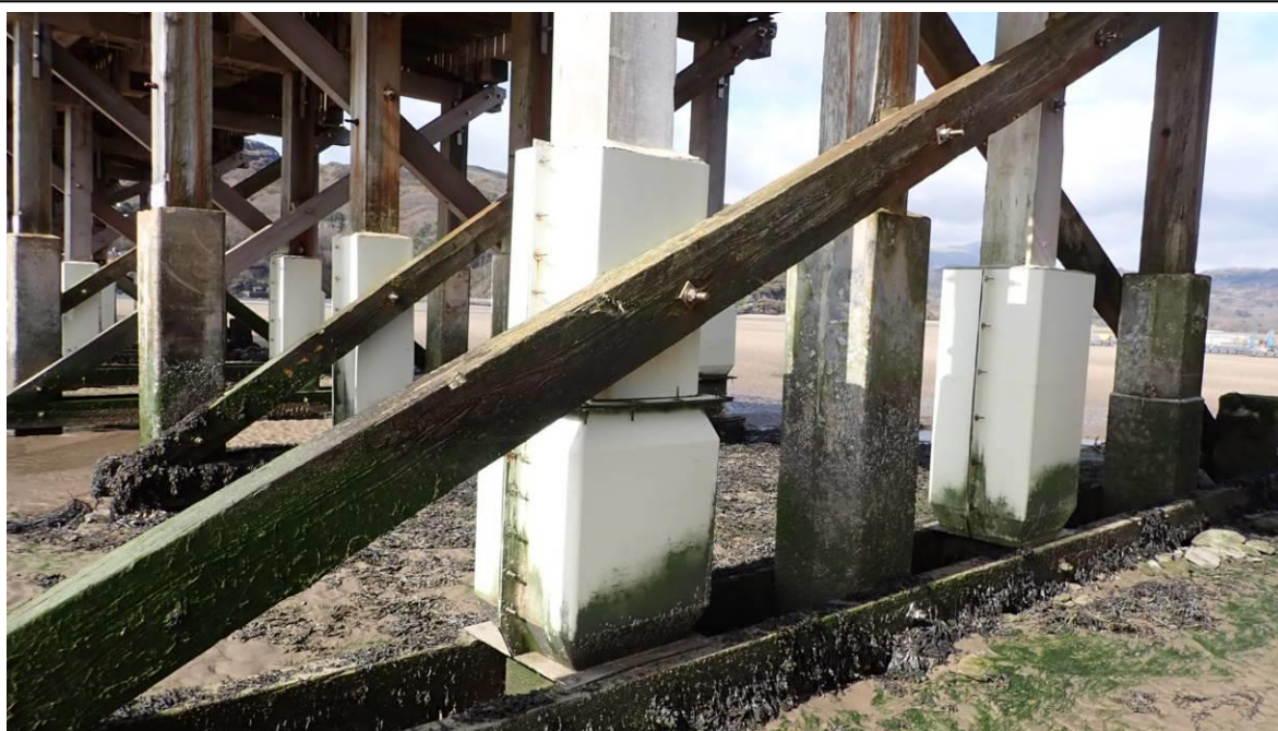
Photo 7 Trestle 2 - Pile 1, new encasement
