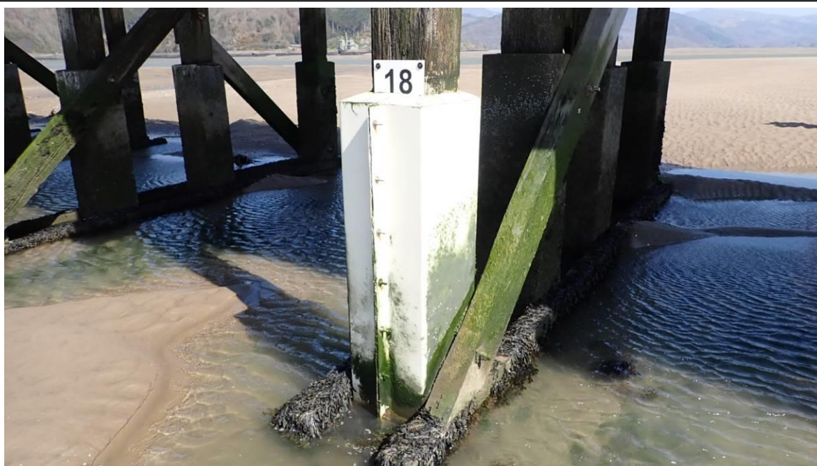
Photo 19 Trestle 18 – Pile 1, new encasement
