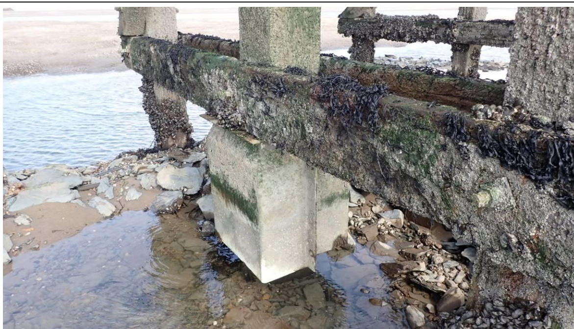
Photo 42 Trestle 93 – Pile 3, New encasement and pile
