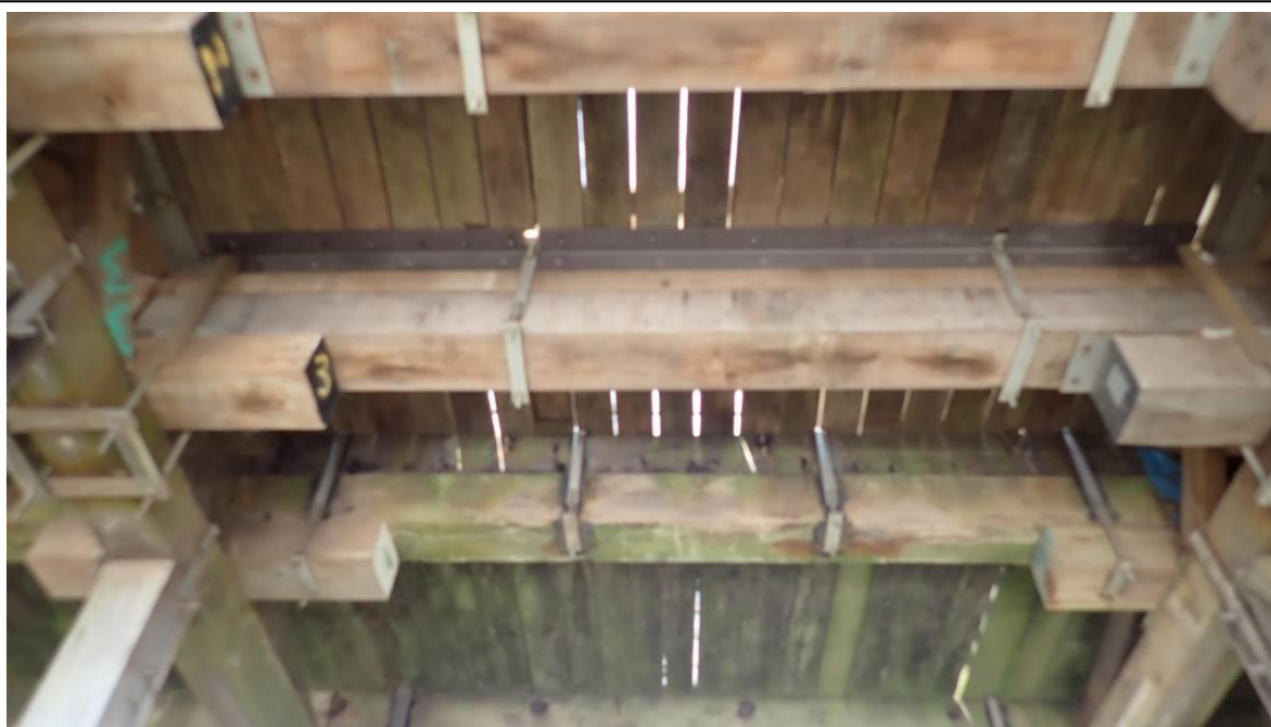
Photo 61 Typical view of the deck
