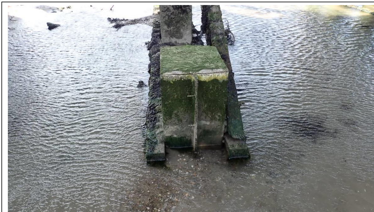
Photo 27 Trestle 27 – Upside outrigger has been repaired
