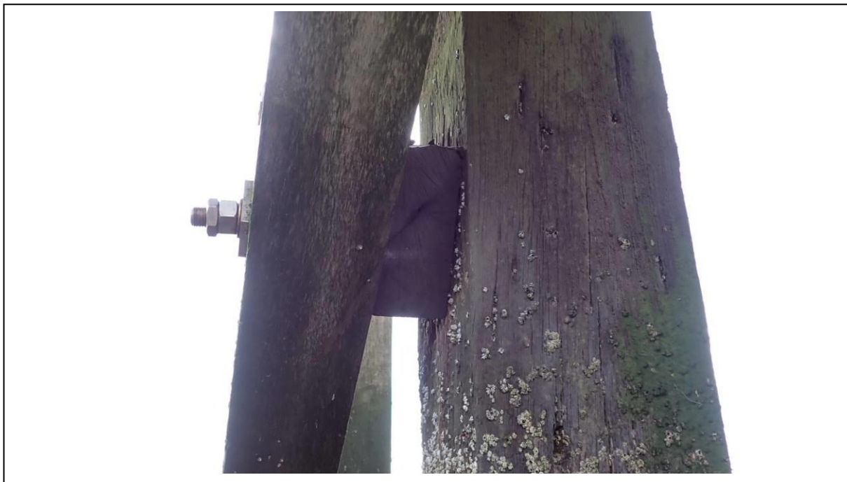
Photo 51 Trestle 73 – New packer installed to LM diagonal brace
