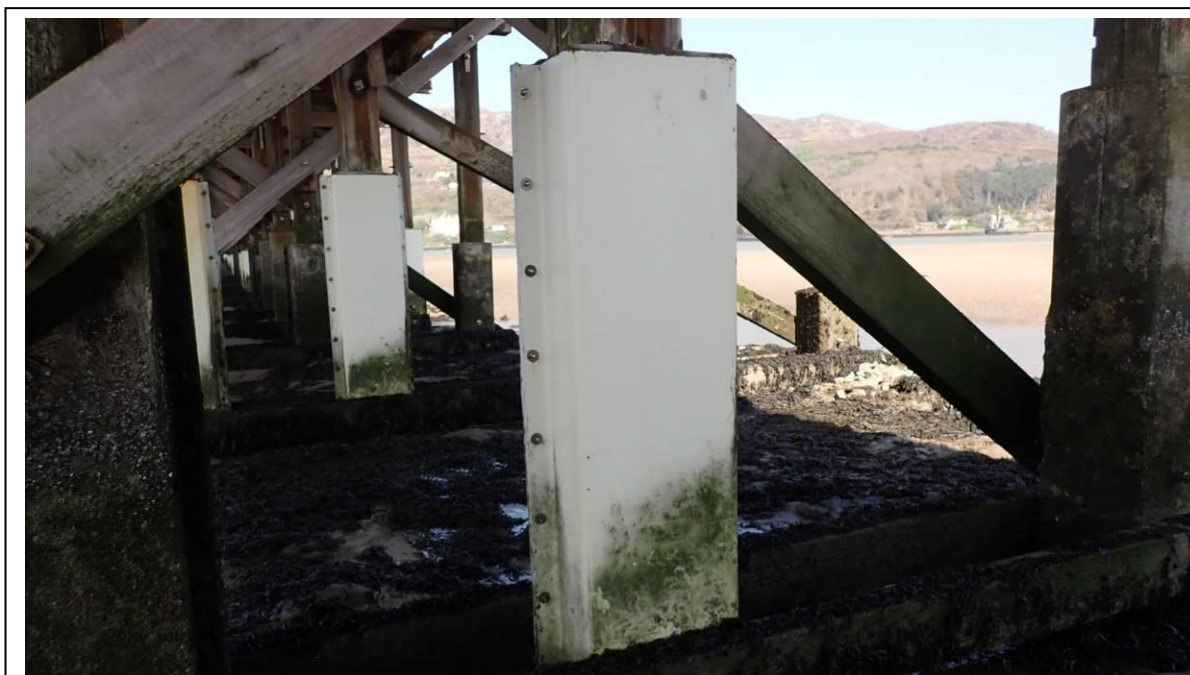
Photo 12 Trestle 6 – Pile 3, new encasement
