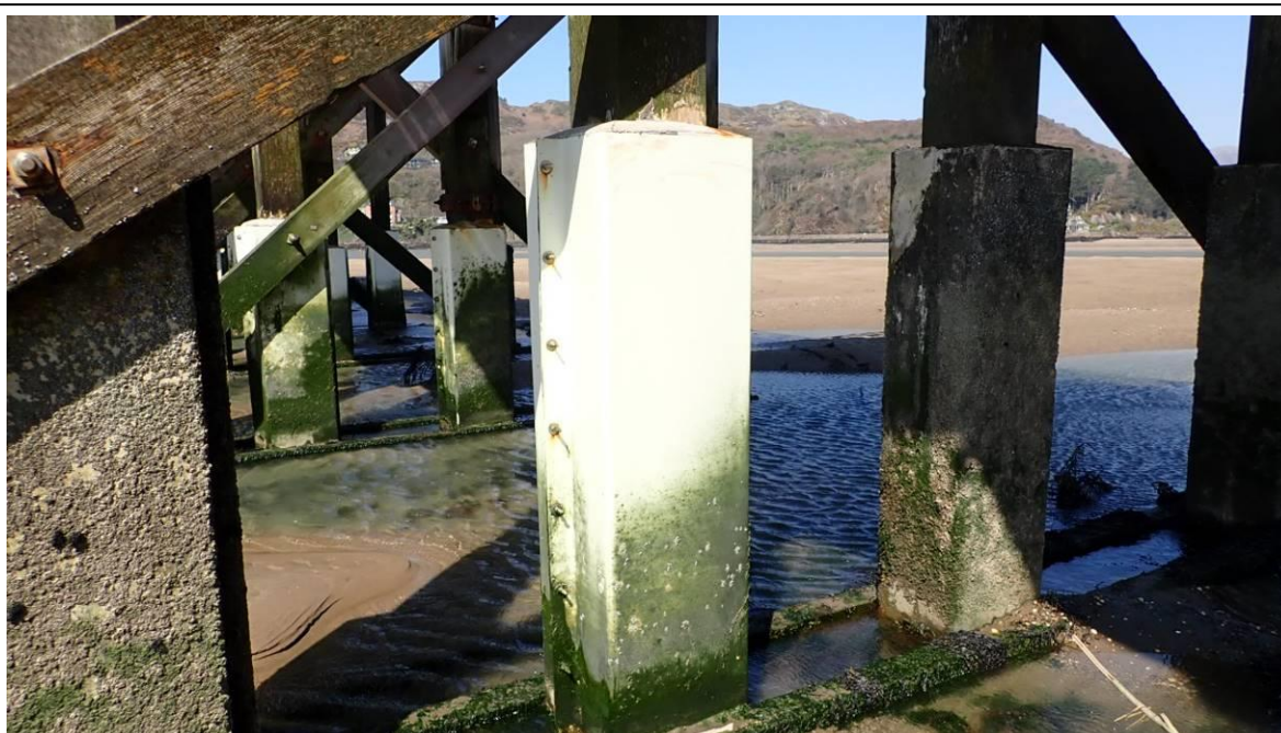
Photo 26 Trestle 27 – Pile 2, new encasement
