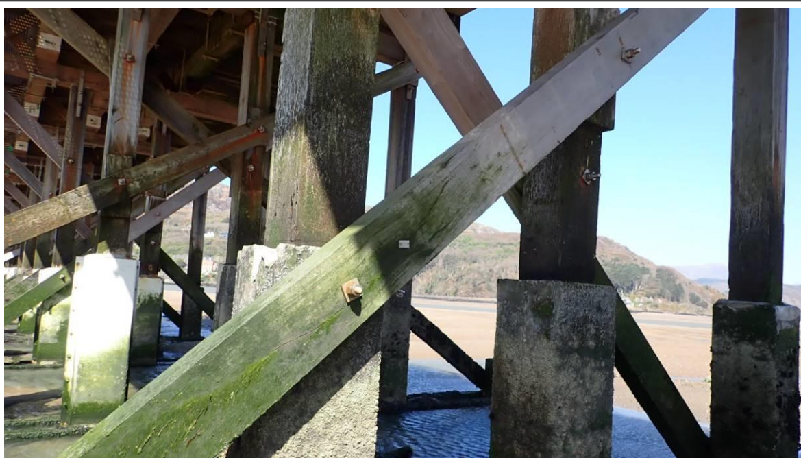
Photo 25 Trestle 26 – NEW LM diagonal brace
