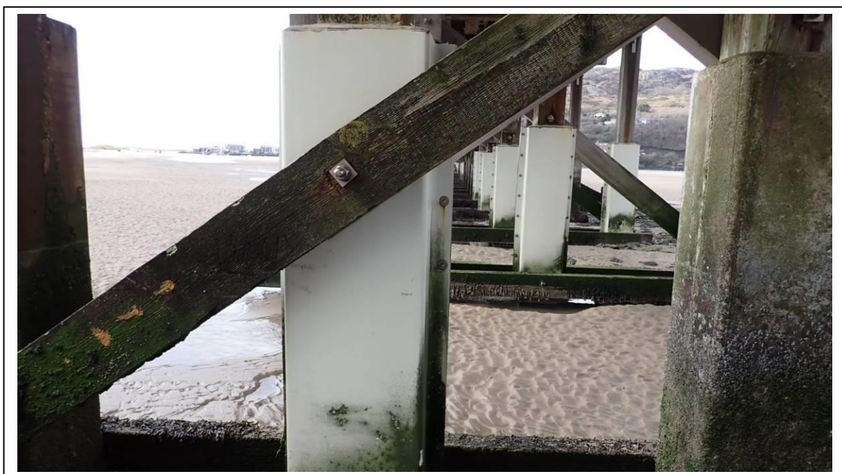
Photo 10 Trestle 10 – Pile 2, new encasement
