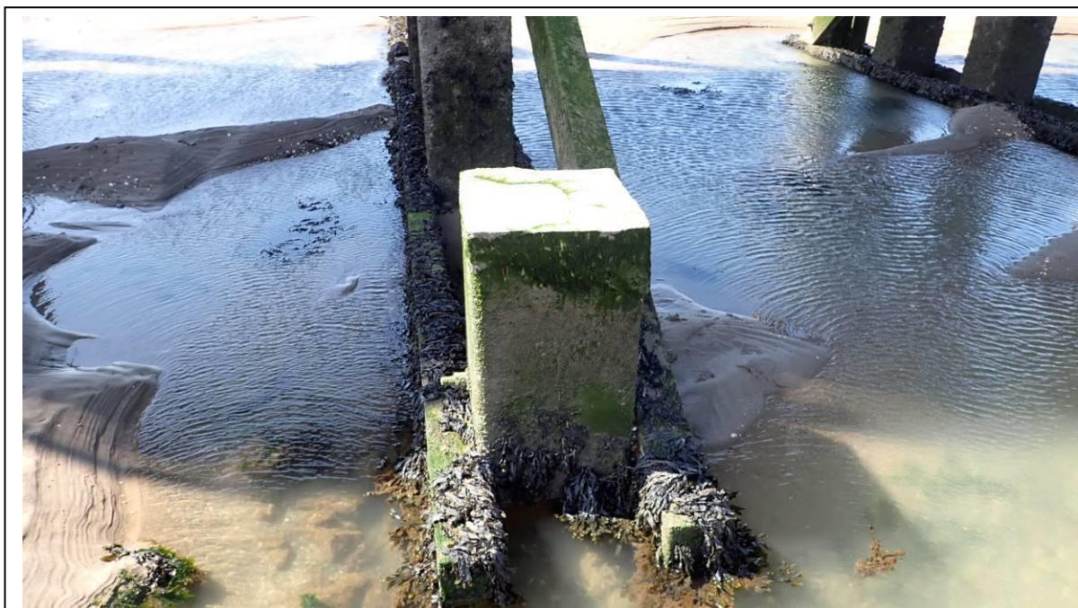
Photo 17 Trestle 17 – Upside outrigger repaired
