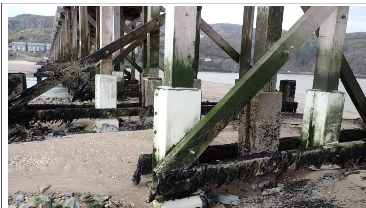
Photo 50 Trestle 71 – Pile 1, new encasement and pile
