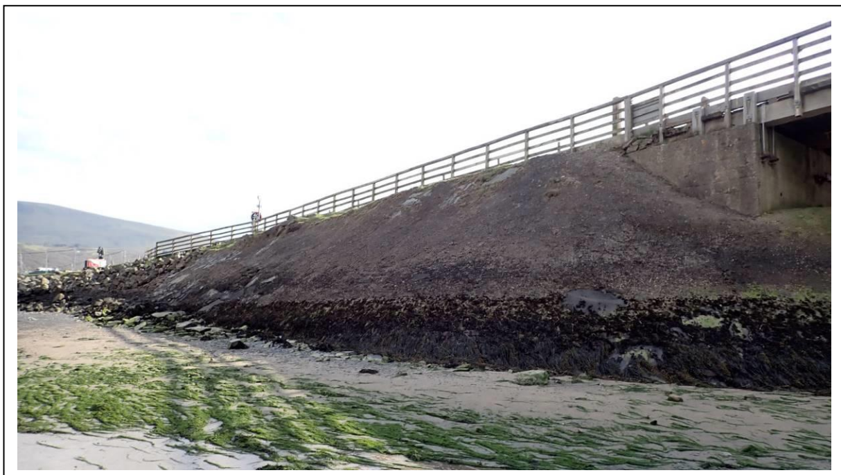
Photo 63 Upstream Low Mileage revetment – separate structure
