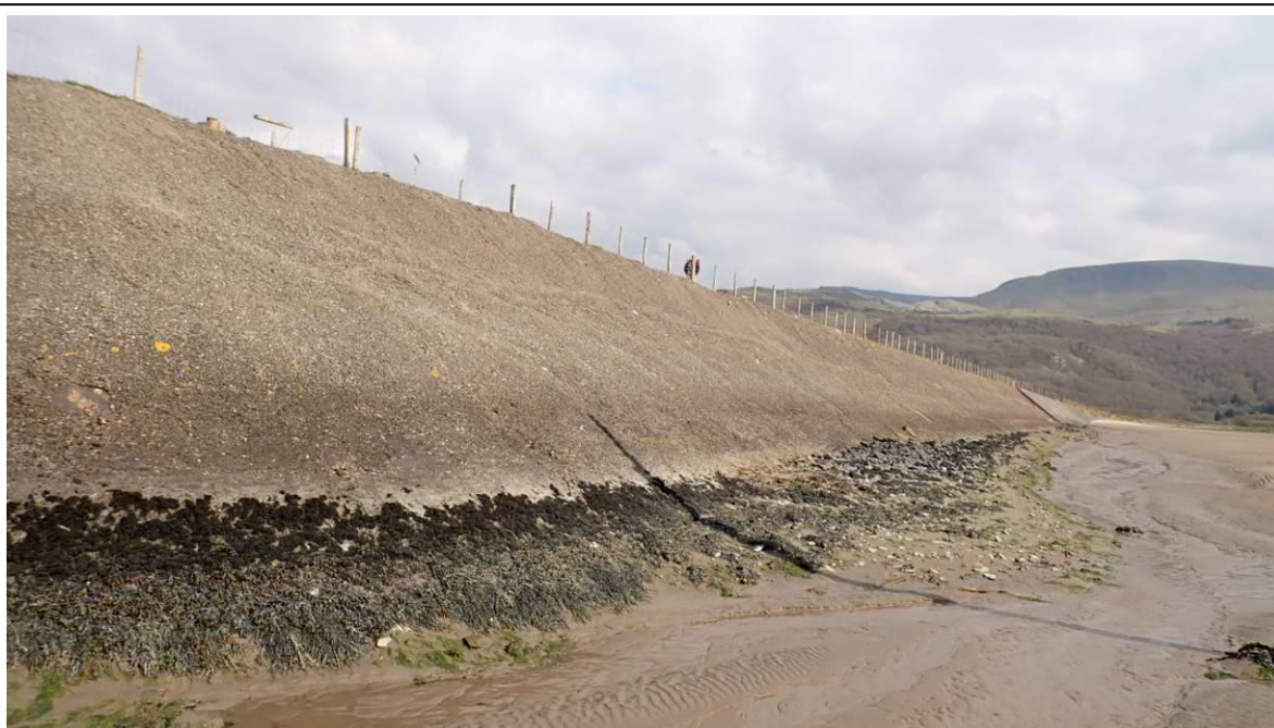
Photo 60 Downstream low mileage concrete revetment – Separate structure
