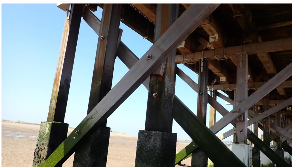
Photo 20 Trestle 20 – New timber to LM diagonal brace, plus new packer
