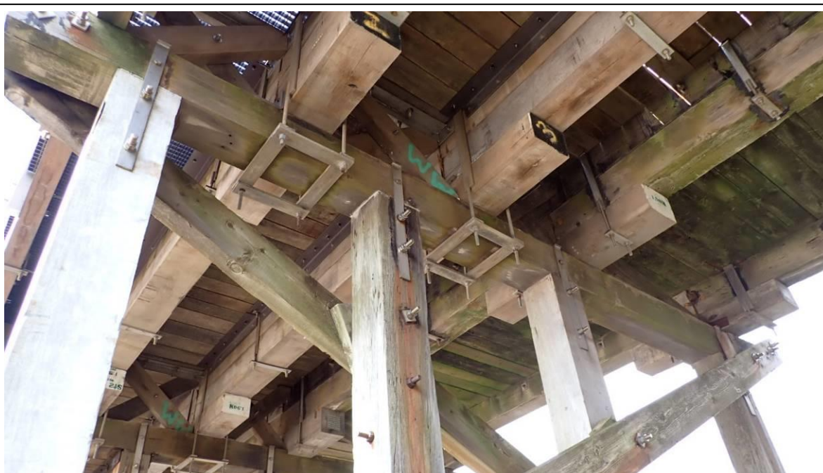
Photo 62 Typical view of cross heads and clamps
