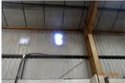
Damaged sandwich panels
