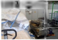
Combustible material in close proximity to electrical installations
