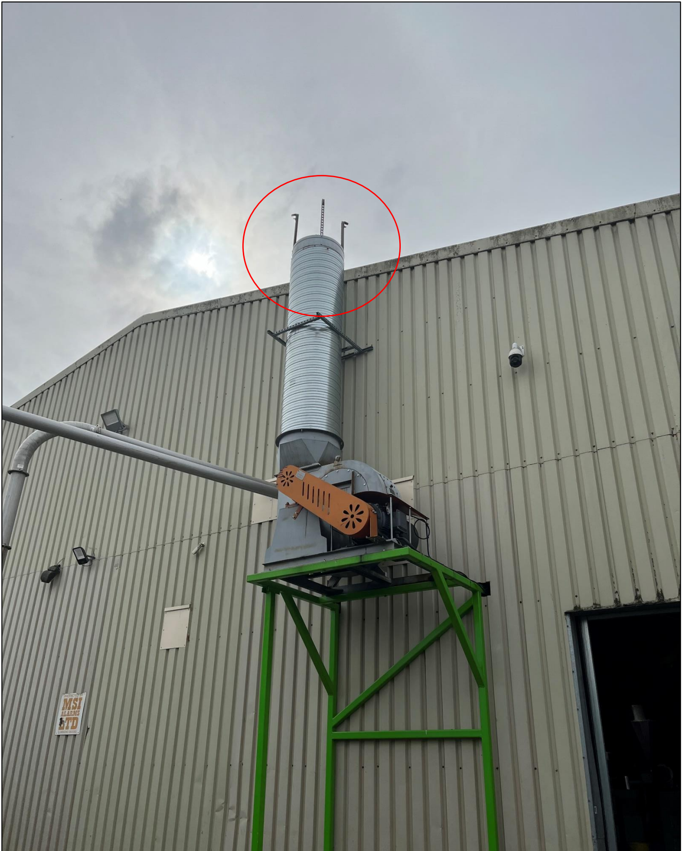
Figure 7: Photograph of the existing building extract fan outlet
