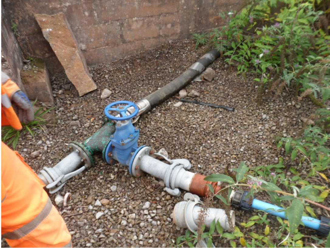
Figure 3 - Image of the Wheel Wash Line Coming off the Main Pump Line (2018)
