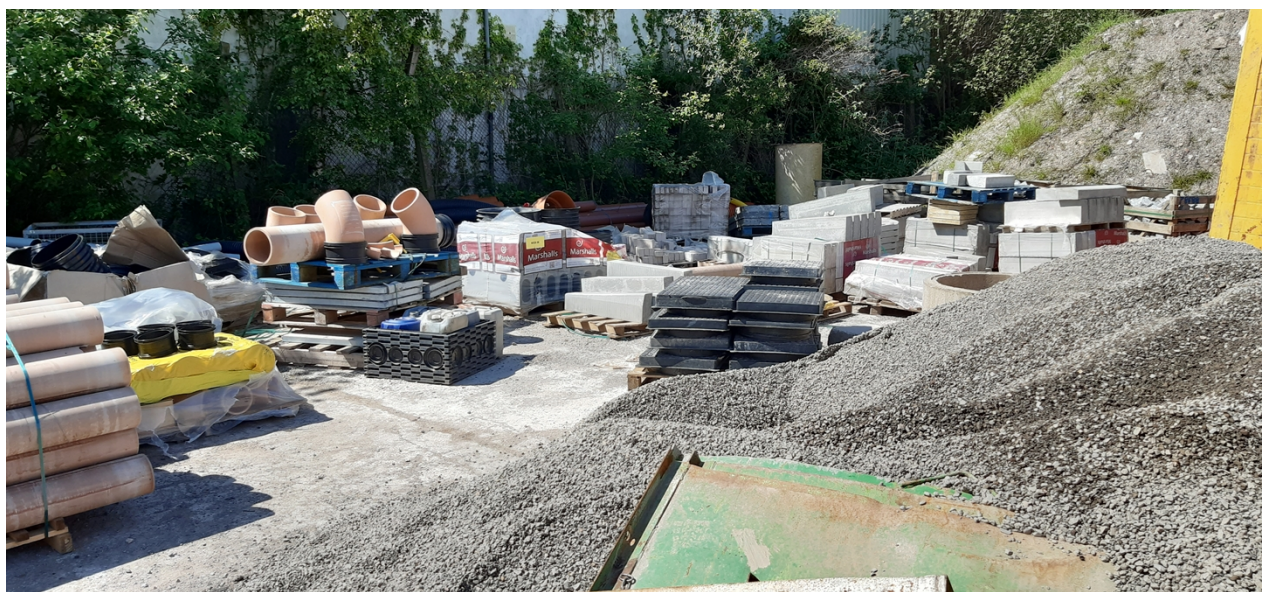
Photo 1 - Overview of site containing building materials
