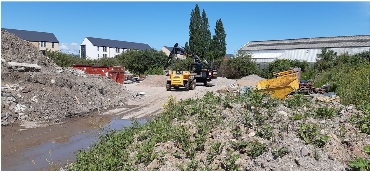
Photo 3 - Overview of site containing soil and rubble
