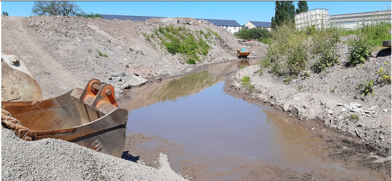
Photo 2 - Overview of site containing soil and rubble
