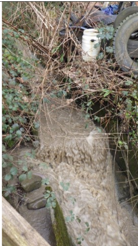
Figure 8 – Site visit photos: Silty water seen flowing at the permitted discharge point at ST2199795988.
