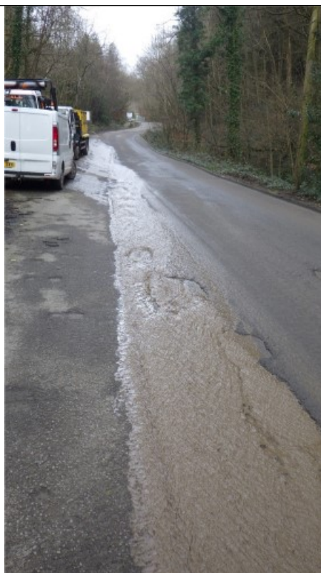
Figure 7 – Site visit photos: Silty runoff seen flowing down Lower Brook Street.
