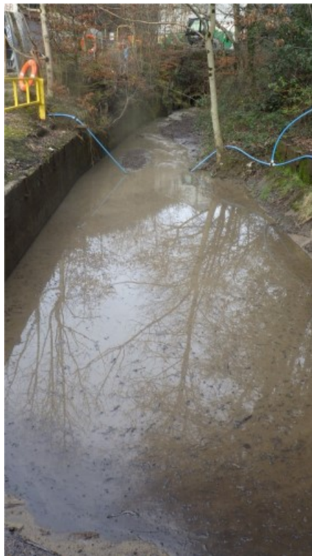
Figure 10 – Site visit photos: The settlement pond at ST2227096357 as observed during the visit. Silt was clearly not settling out before discharging off site.
