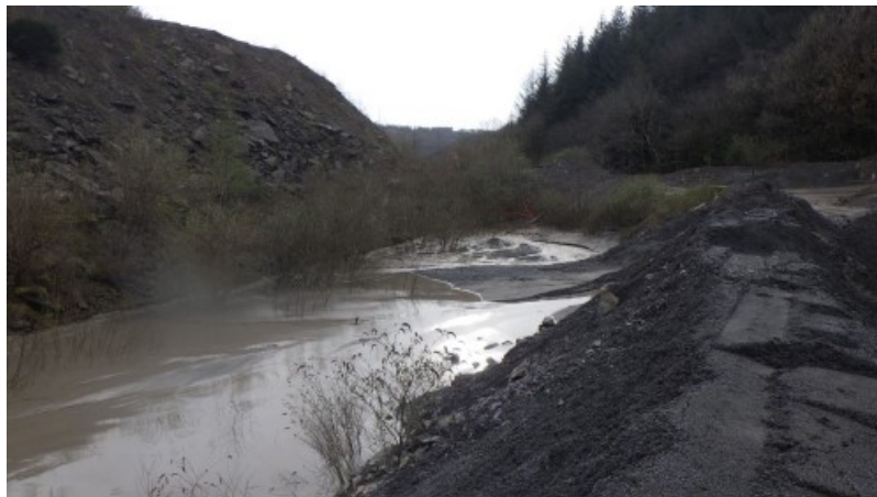
Figure 17 – Site visit photos: Settlement pond 1 as observed during the visit from ST2257396557. Active pumping from settlement pond 2 into settlement pond 1 is visible here.
