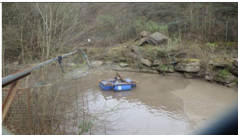
Figure 20 – Site visit photos: Settlement pond 2 as observed during the visit from ST2243496478. Pumping operations are seen here, which were noted to have been taking place on site for “a long time.”
