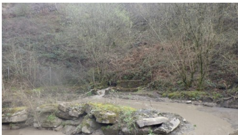
Figure 21 – Site visit photos: Settlement pond 2 as observed during the visit from ST2243496478. The point where the discharge from pond 1 enters pond 2 can be seen here.
