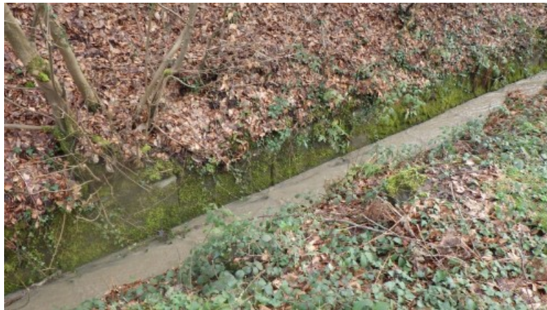
Figure 15 - Site visit photos: The silty discharge observed leaving site and into the concrete channel at ST2223596317.
