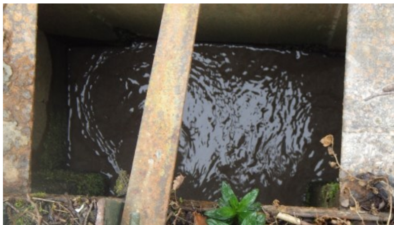
Figure 11 – Site visit photos: Silty water seen exiting the settlement pond at ST2227096357.
