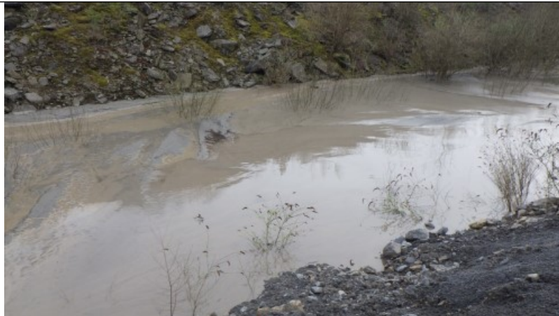
Figure 18 – Site visit photos: Settlement pond 1 as observed during the visit from ST2257396557. The water appears heavily silted throughout.
