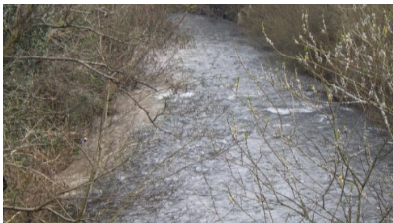
Figure 4 – Site visit photos: Downstream view of the main river from the road bridge at ST2164295798. Brown discharge seen entering the watercourse from Nant Hafod-fach ~100m downstream of this point at ST2165995732.
