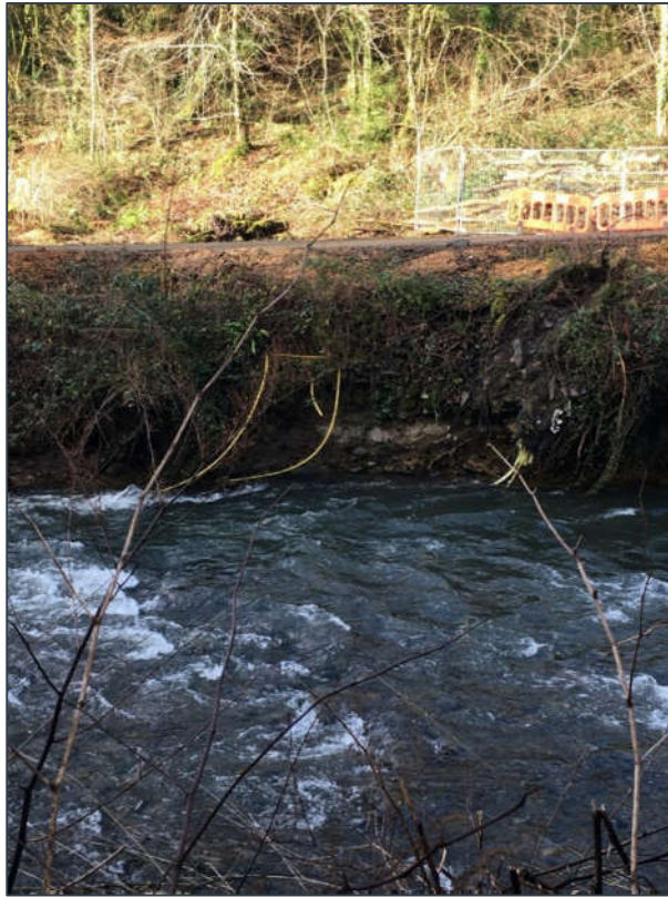
Figure 6 - Ongoing Riverbank erosion exposing made ground and stone buttress (Winter 2023/24)
