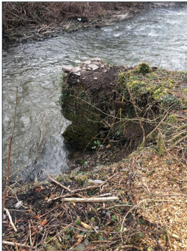
Figure 7 - Exposed stone buttress and ongoing erosion (low water winter conditions Winter 2023/24)
