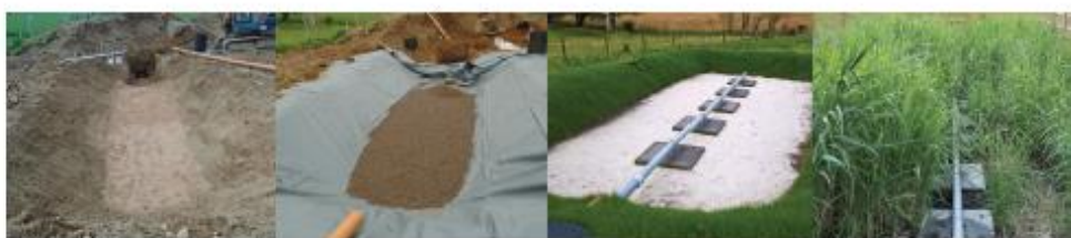
Sequence of activities in wetland construction. Photo courtesy of Moir Environmental
