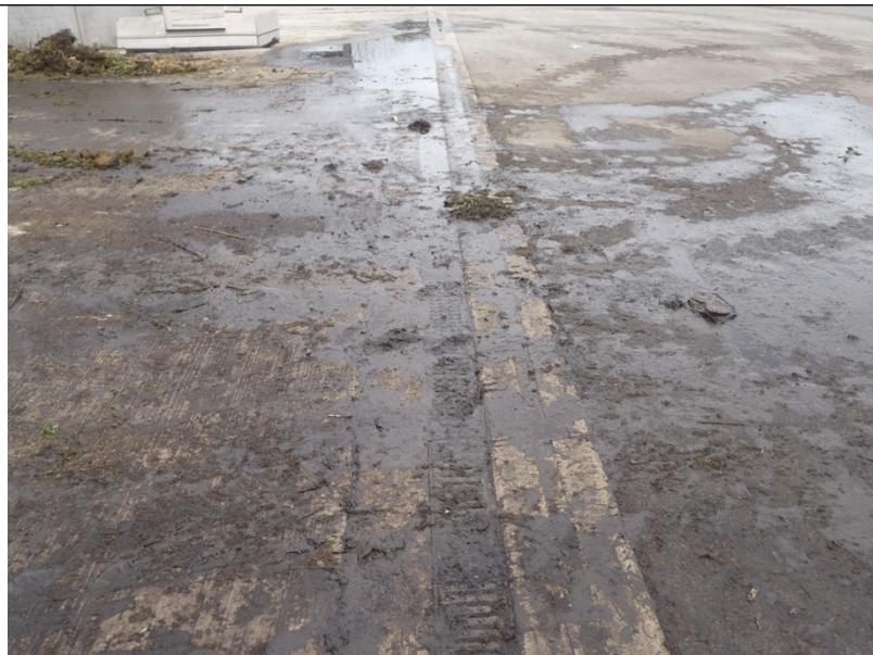
Blocked drain in front of green waste bay
