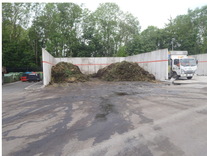
Contaminated water being tracked across yard
