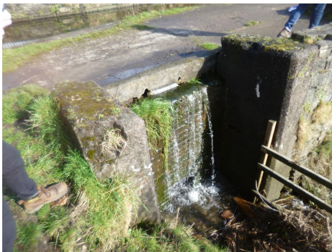
Photo 3: Existing spillway/weir from Tennant Canal to River Clydach (Clydach Aquaduct on Tennant, reference 82339)
