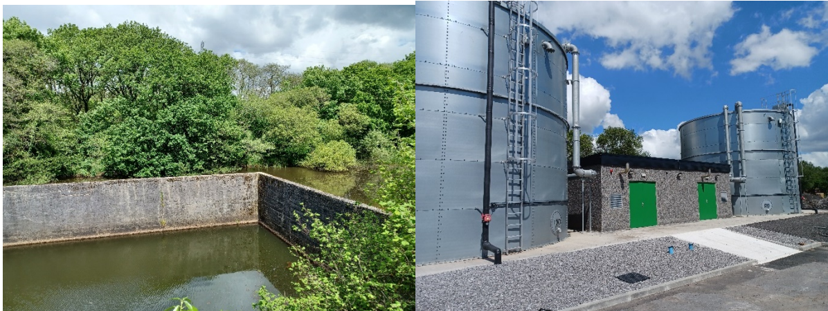
Lagoon shown on left and sprinkler tank system shown on right
