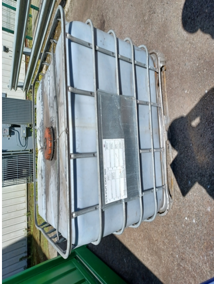
IBC without secondary containment
