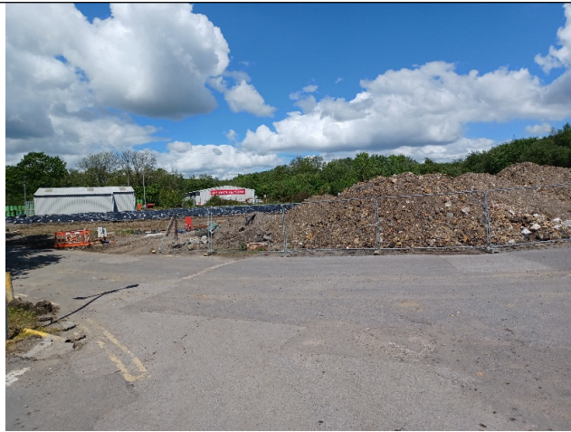
Construction works for new building and car park
