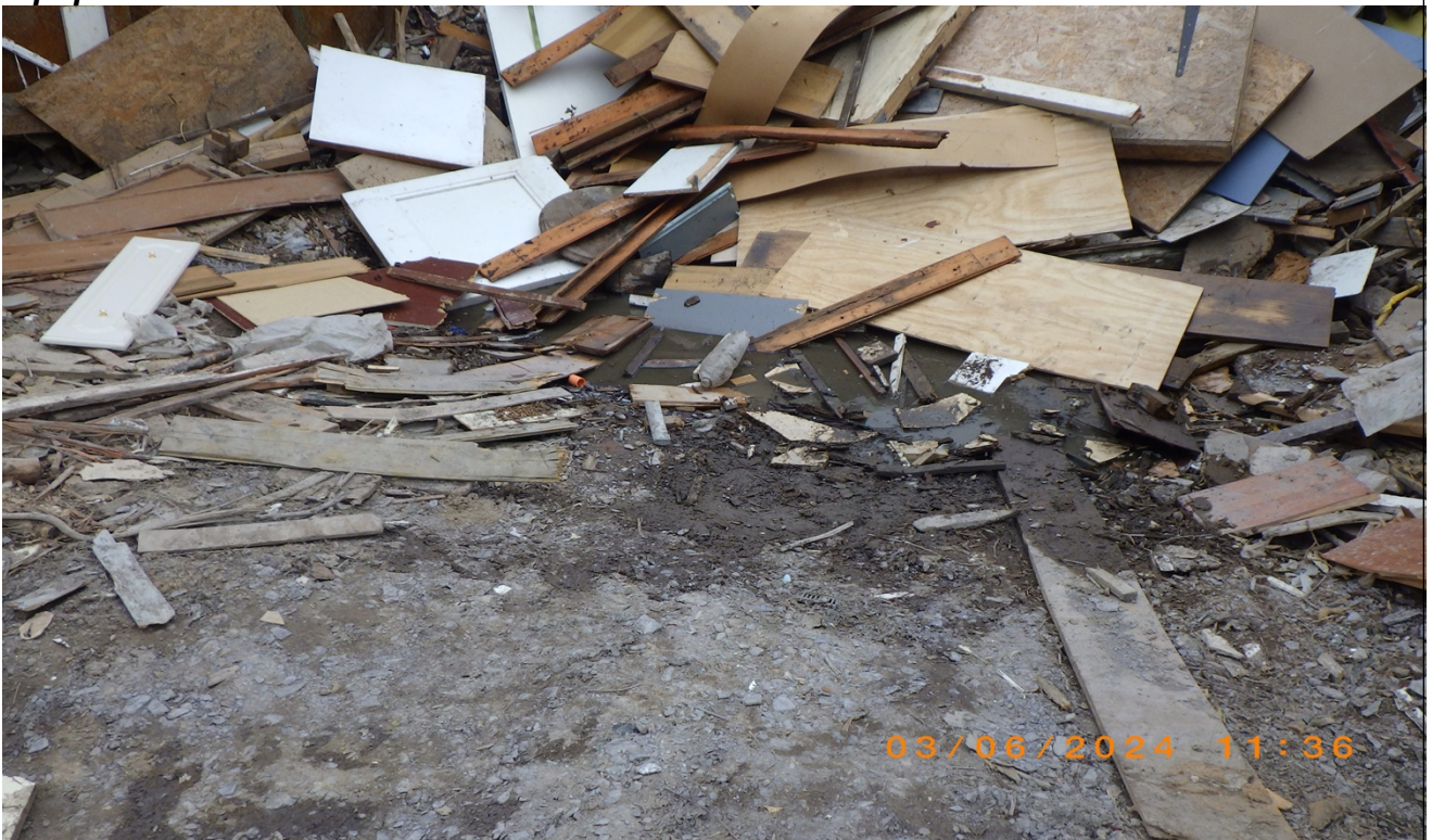
Photograph showing storage of combustible wastes on permeable ground
