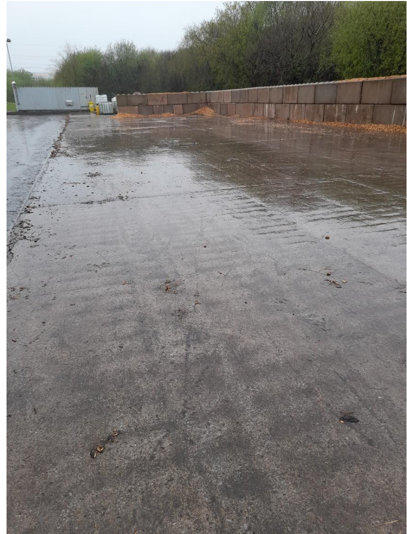
Figure 4 – Condition of existing impermeable concrete pad (central and western end).
