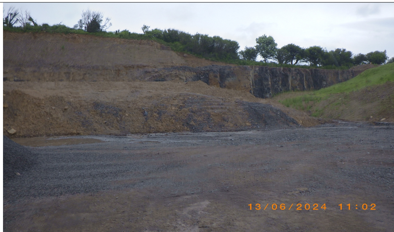
Photograph showing excavated material from site and location of new landfill cell
