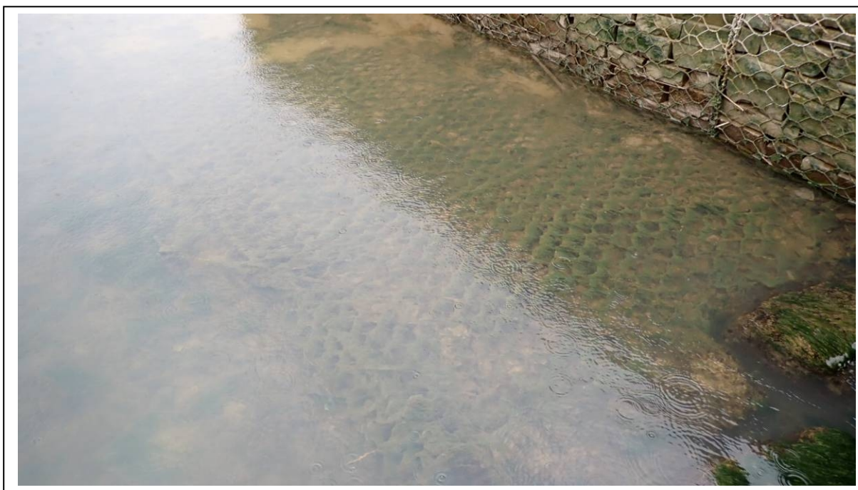
Photo 4 Gabion bed basket fronting upside low mileage training wall
