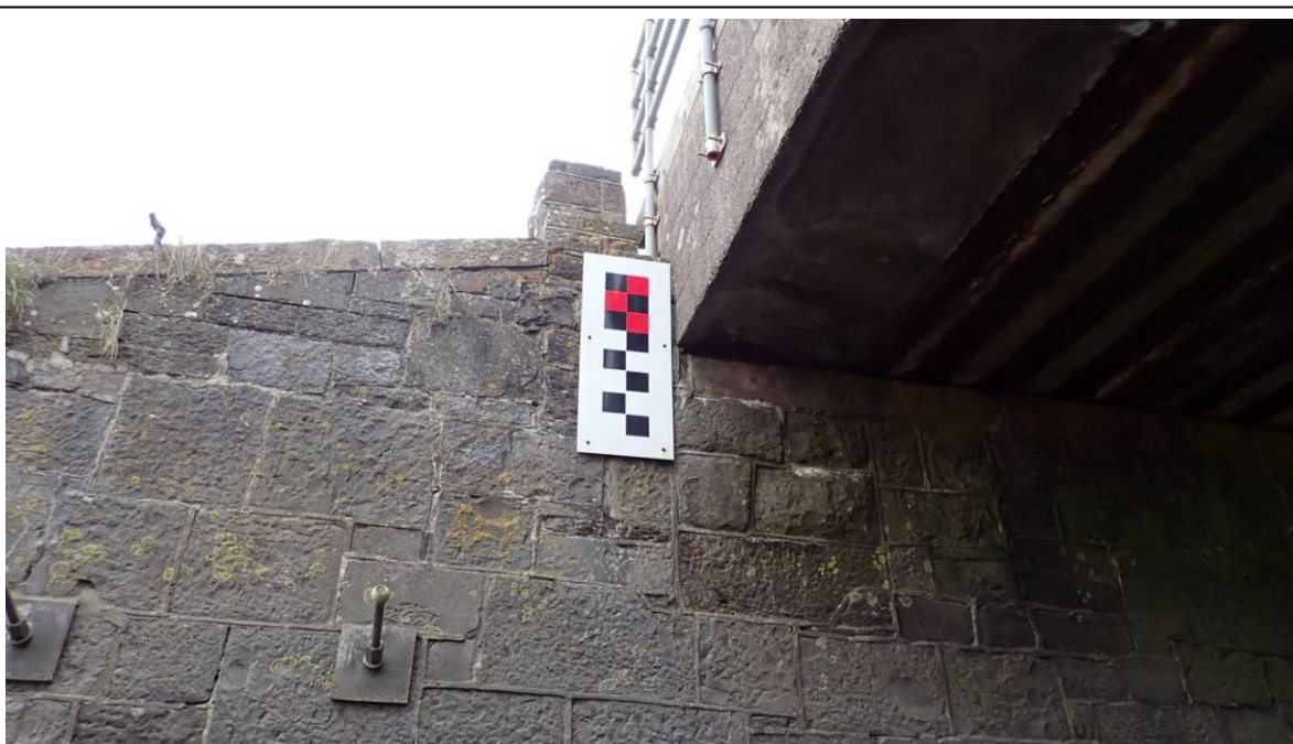
Photo 28 View of flood board
