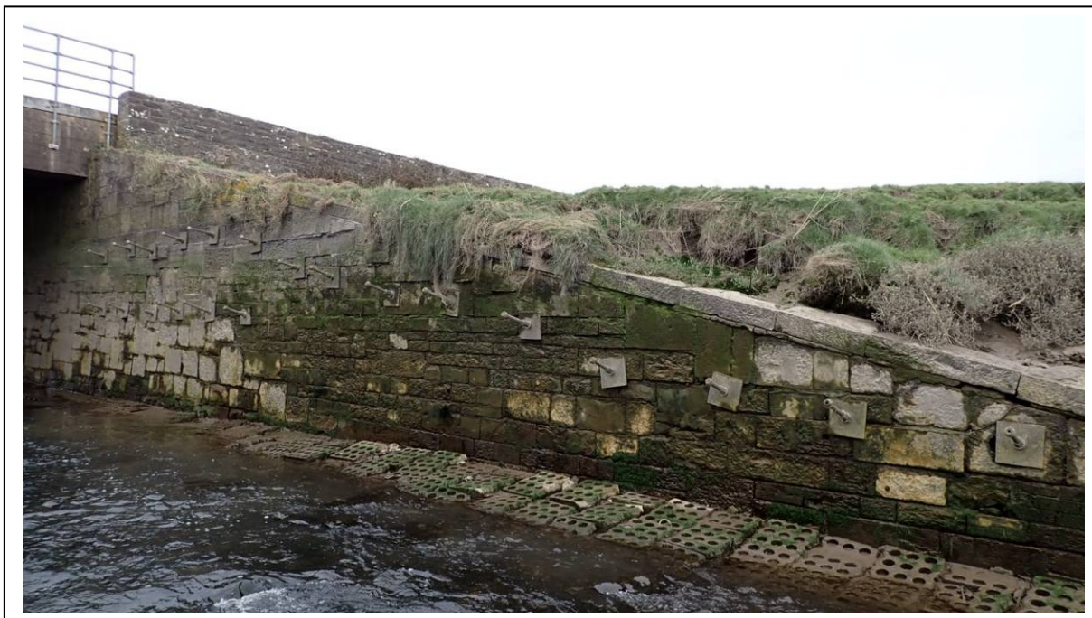
Photo 19 Downside low mileage wingwall
