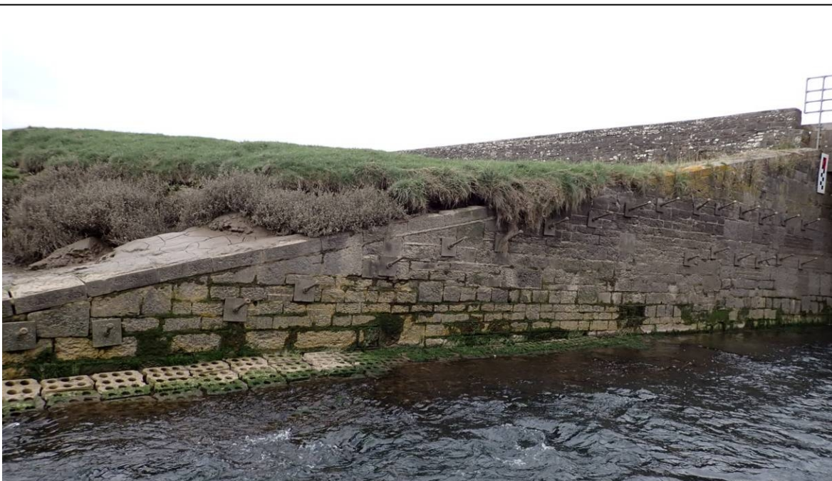
Photo 22 Downside high mileage wingwall
