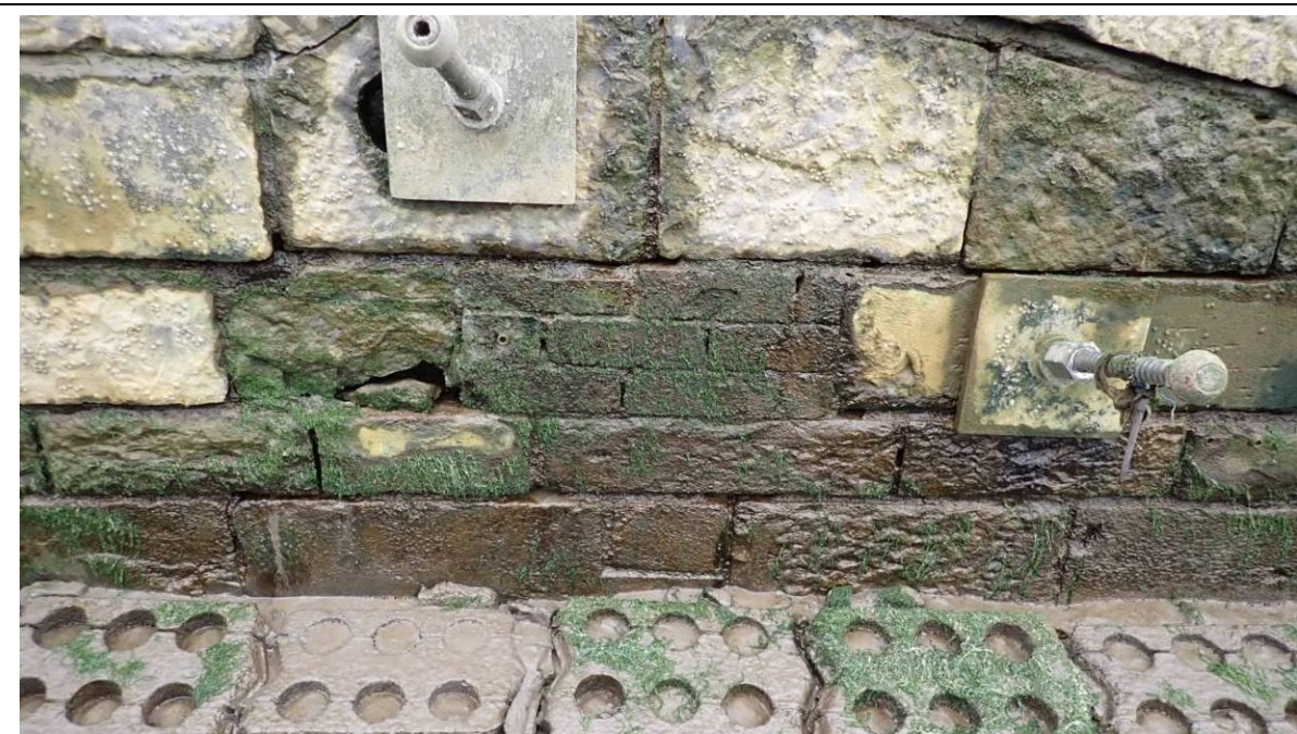
Photo 20 Open joints
