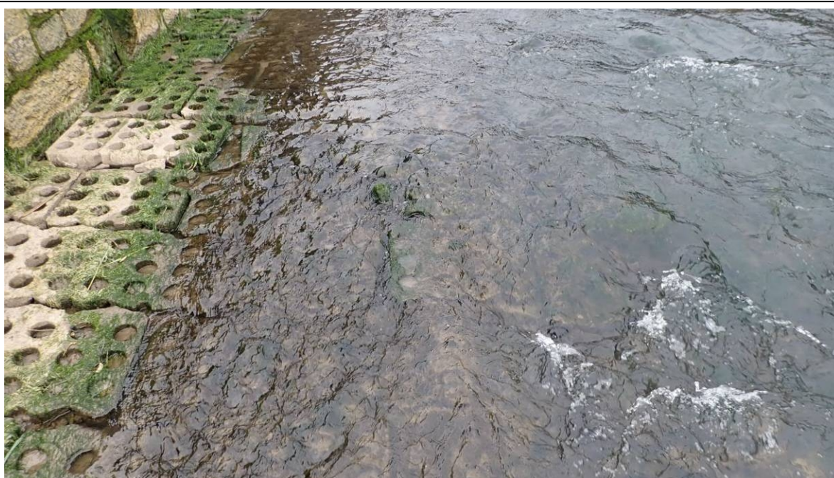
Photo 24 Typical view of invert
