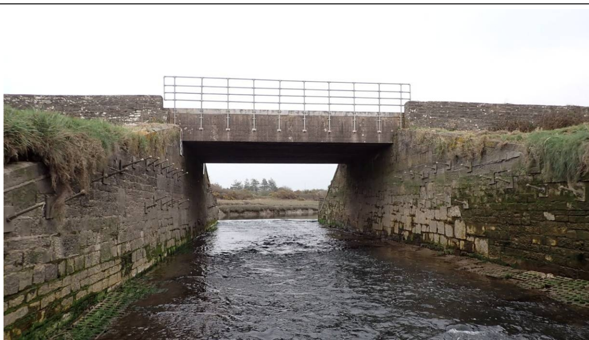
Photo 26 Downside / downstream elevation
