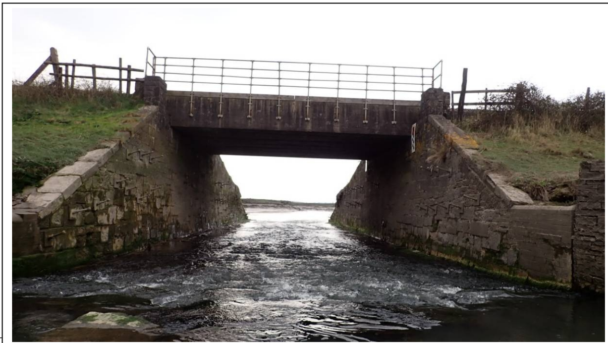
Photo 1 Upside / upstream elevation
