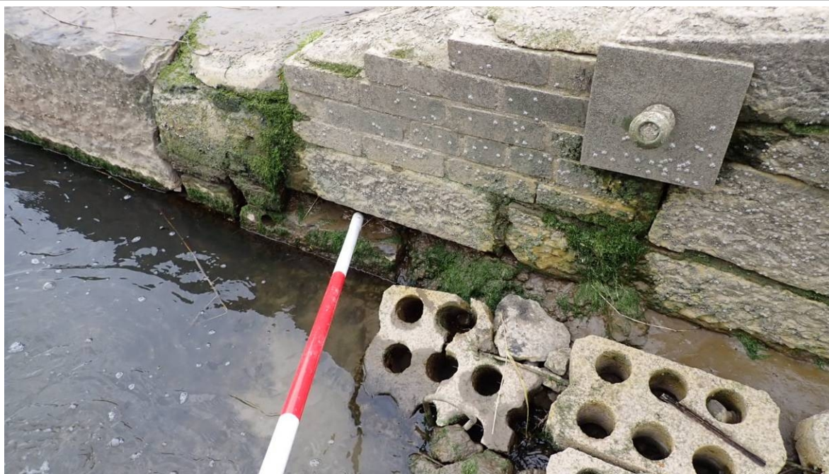
Photo 23 Void to downstream end
