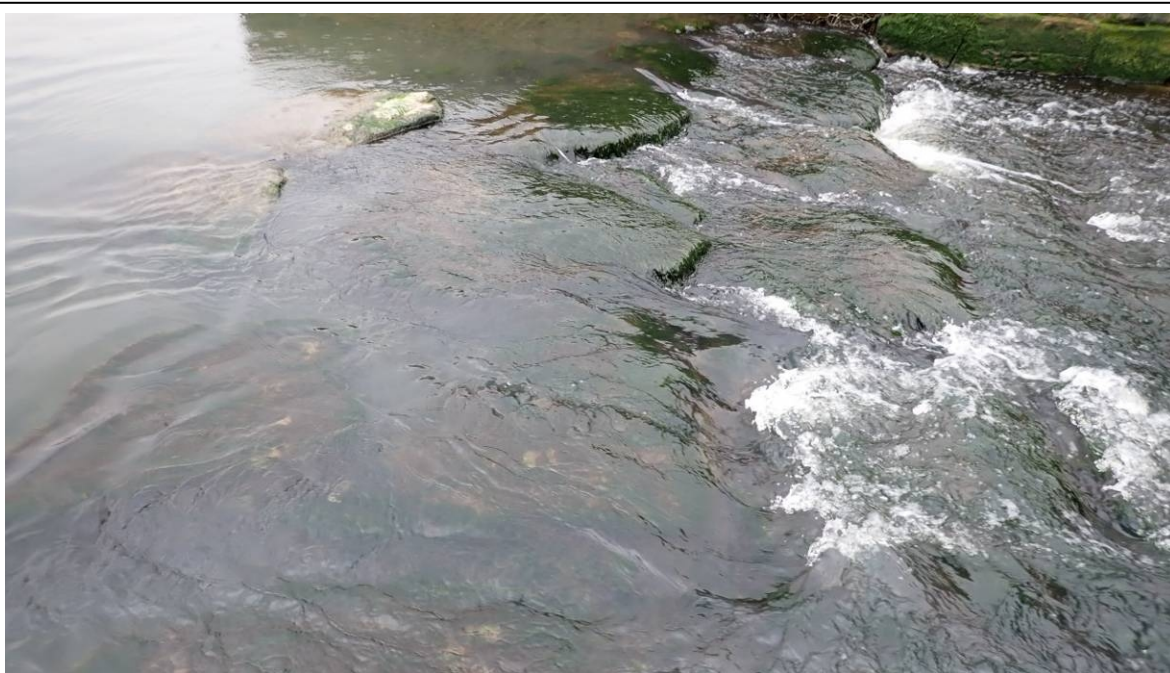
Photo 7 Rock armour to upstream end of invert
