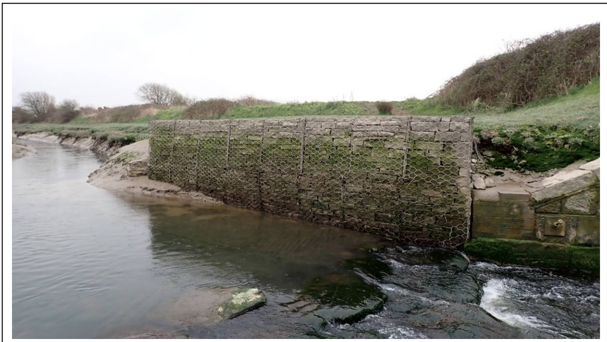
Photo 3 Upside low mileage gabion training wall
