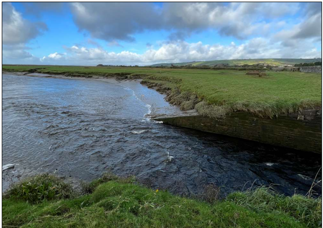
Figure 4: Downstream side of the structure flowing into the wider estuary.
