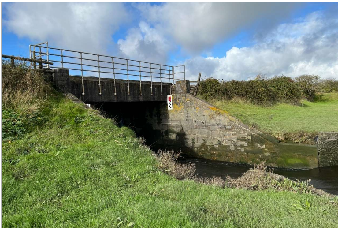
Figure 1: Upstream view of structure.
