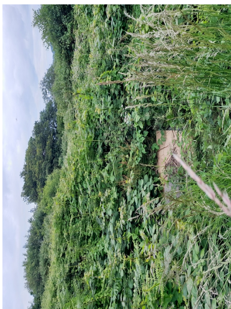
Hardboard covering access chamber, drainage field over grown.
