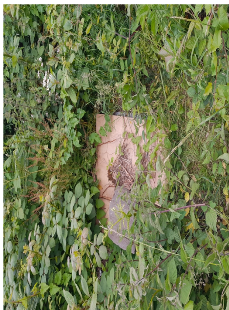
Hardboard covering access chamber, drainage field over grown.
