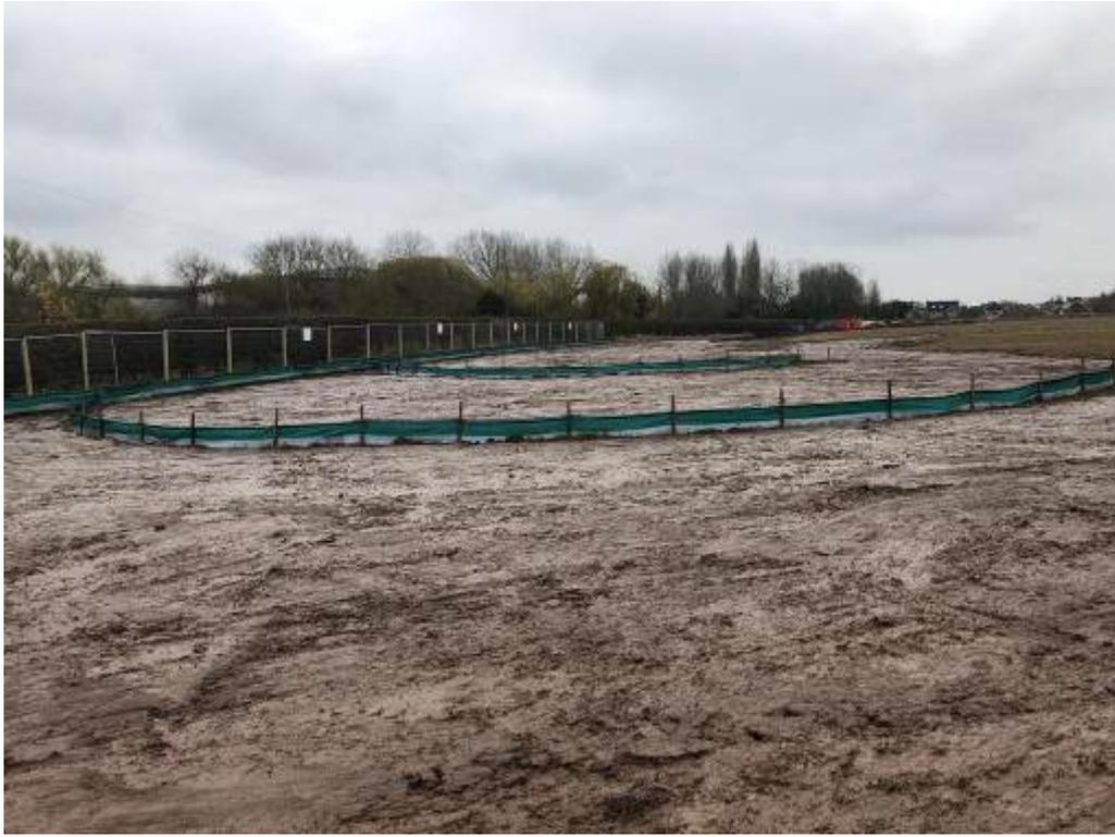
Placement of silt matting to capture settled silt downgradient within a surface watercourse
