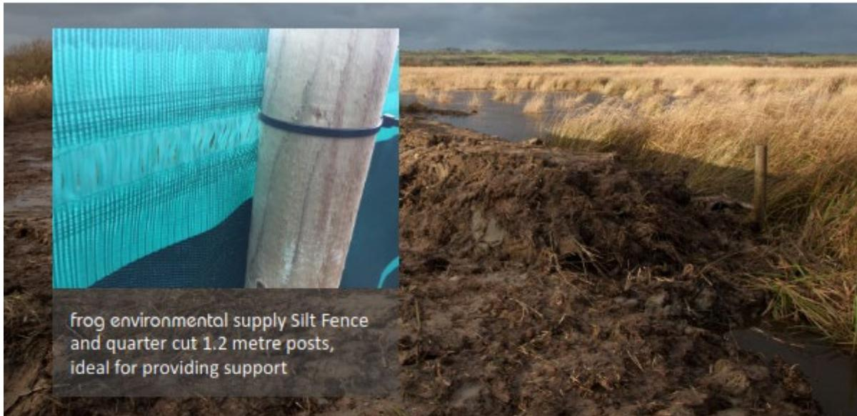
Silt Fence is inexpensive to buy and install, but it must be correctly positioned and maintained for it to be an effective pollution control measure.
