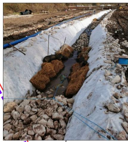
Cut off ditch: consider adding Floc Mats™ along with the Silt Mats™. Each set should contain 6 mats in a ratio of 1:1. First, install the Floc Mats™ upstream followed by the check dam, then the Silt Mats™. Repeat this sets every 10 metres upstream, then space them out more towards the discharge location.
