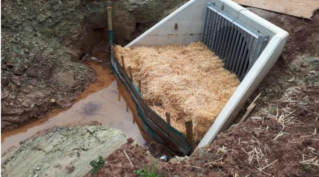
Silt fencing installed across an outfall headwall, to promote settlement of silt within the concrete apron prior to discharge into the surface watercourse (in the event of breach of other control measures)
