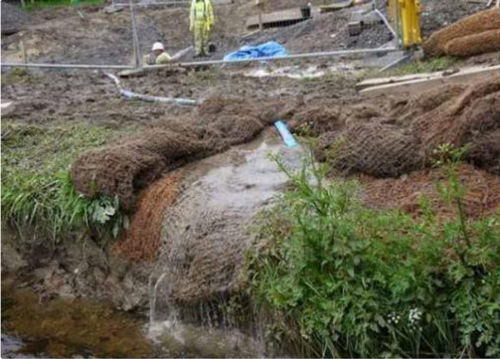
Silt Wattles utilised to separate clean and silty water within a watercourse
