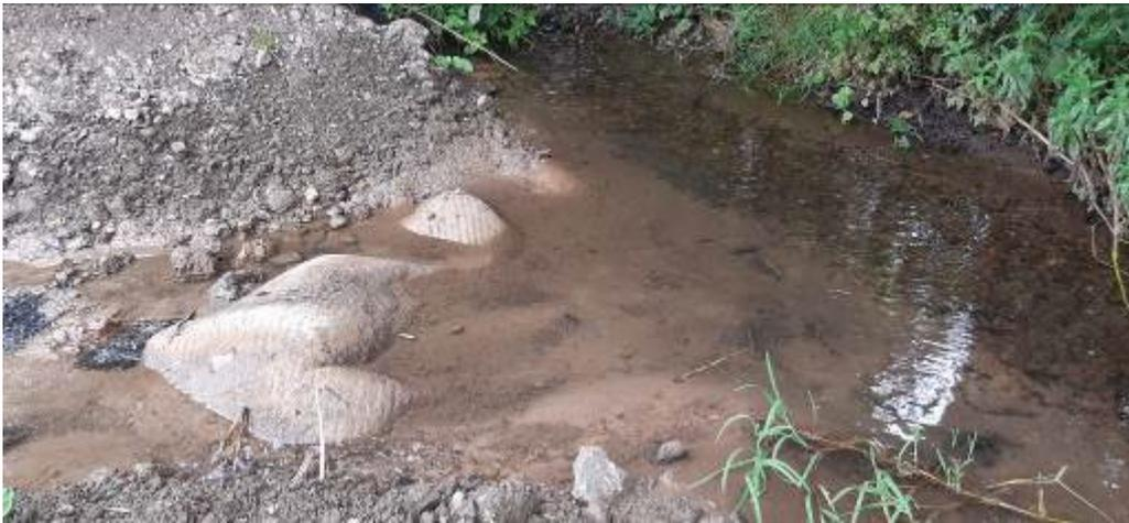
Dewatering bag used to treat water pumped from excavations. Dewatering bag is placed upon a pallet for ease of movement, onto clean gravel to dissipate the flow and prevent scouring, in a vegetated area for infiltration.
