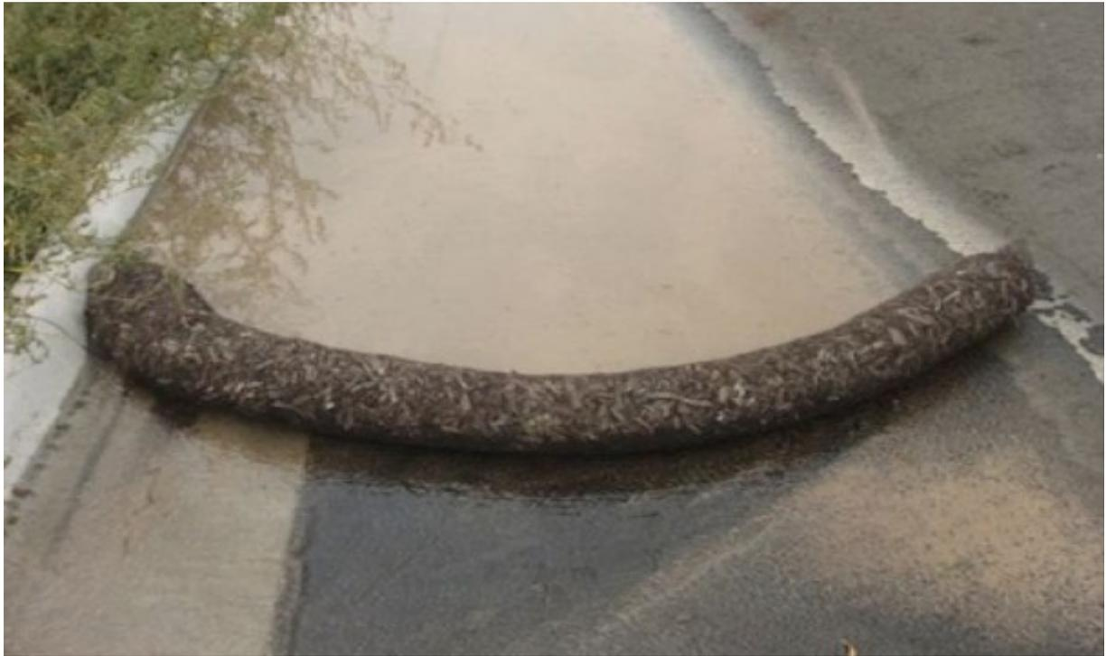
Silt matting and Silt Wattles deployed within a surface watercourse. Silt Wattles create a check dam promoting settlement of suspended solids, which is captured by the silt matting.
