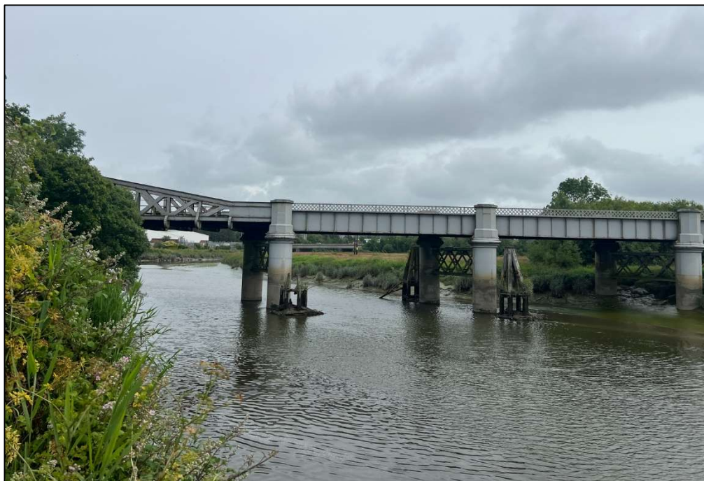
Figure 2: View of swing bridge and timber fenders (Downstream of structure).
