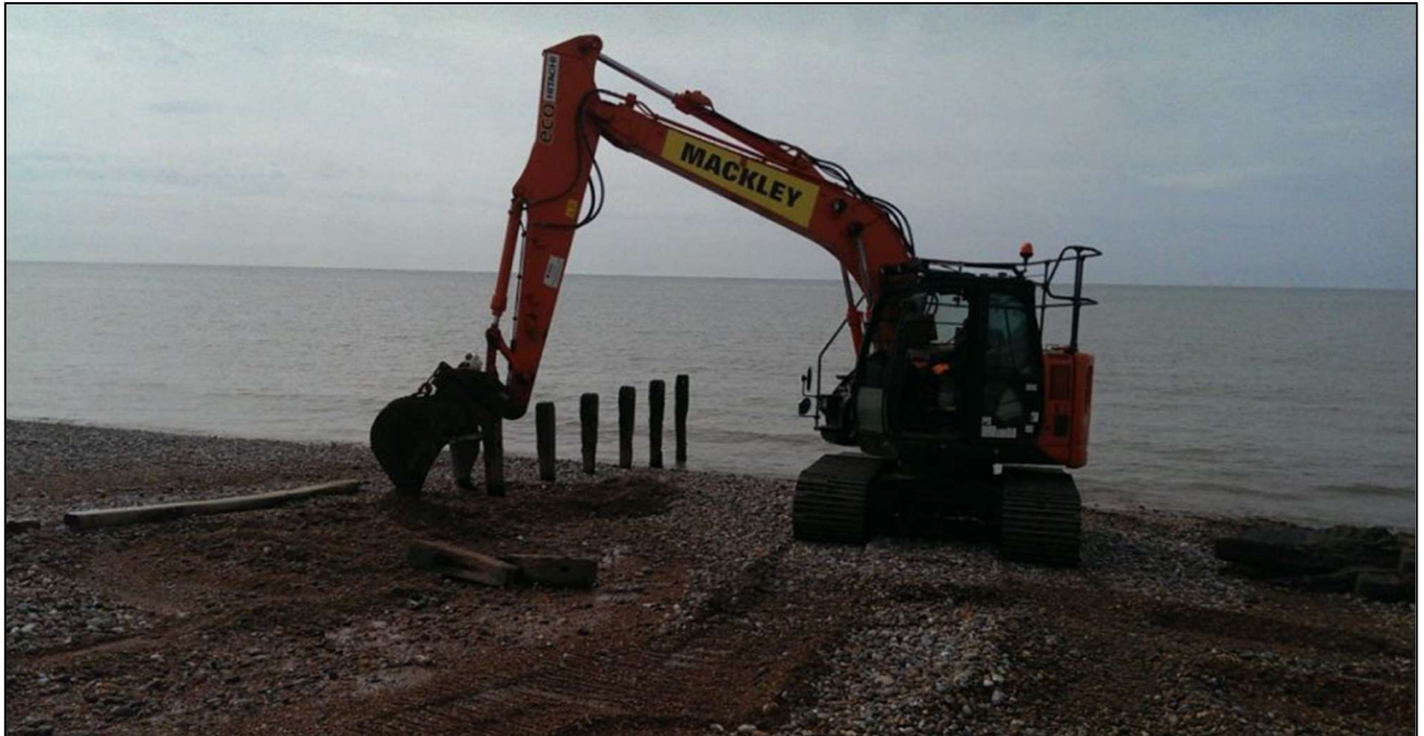
Figure 5: Example of similar tonne excavator removing timber groynes.
