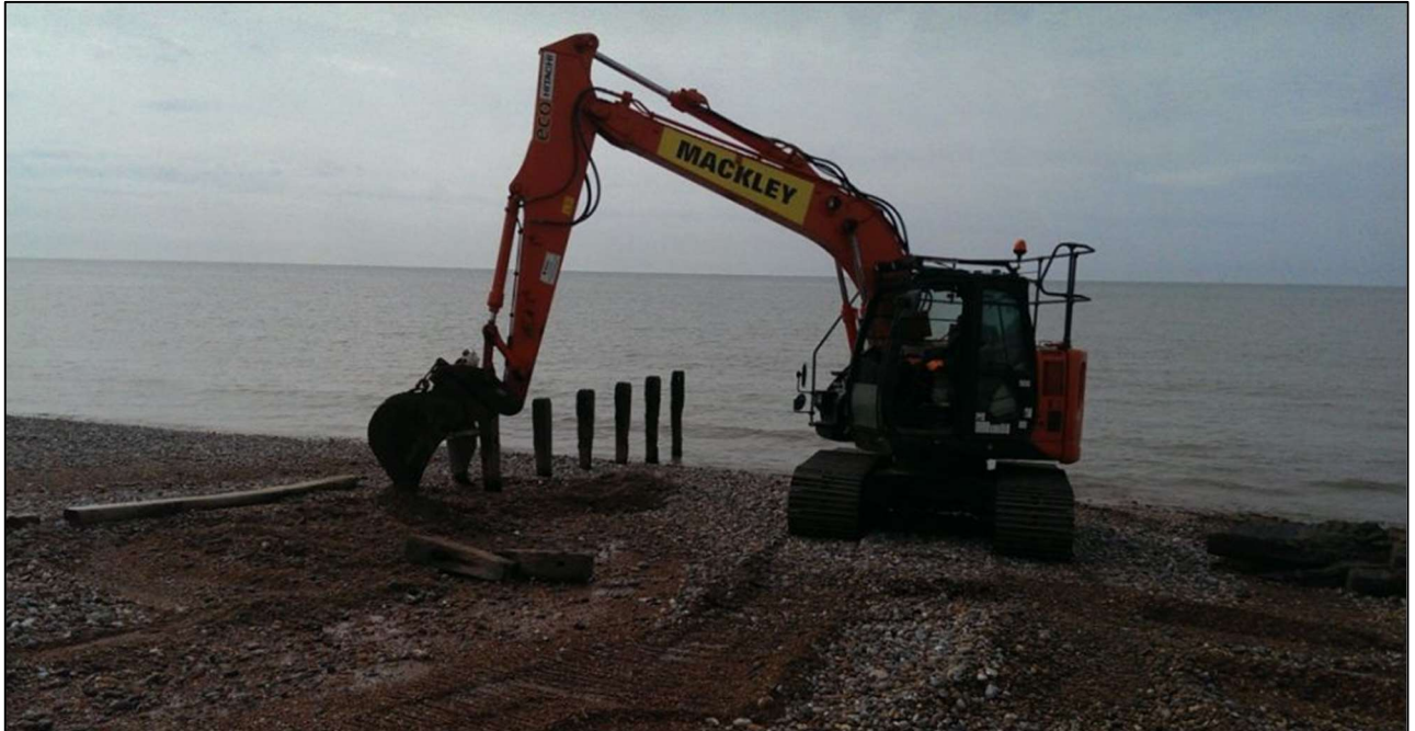
Figure 4: Example of similar tonne excavator removing timber groynes.
