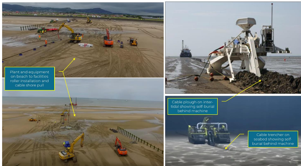
Figure 1.1: Typical Plant And Equipment For Cable Installation Across Inter-Tidal Similar To Cable Historically Installed Between Prestatyn And Rhyl.
