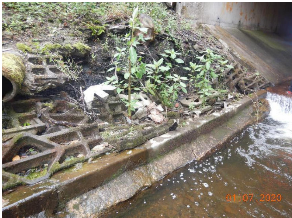
Photo 74 – Failed revetment resulting in embankment scour (139.7m – 143.7m)
