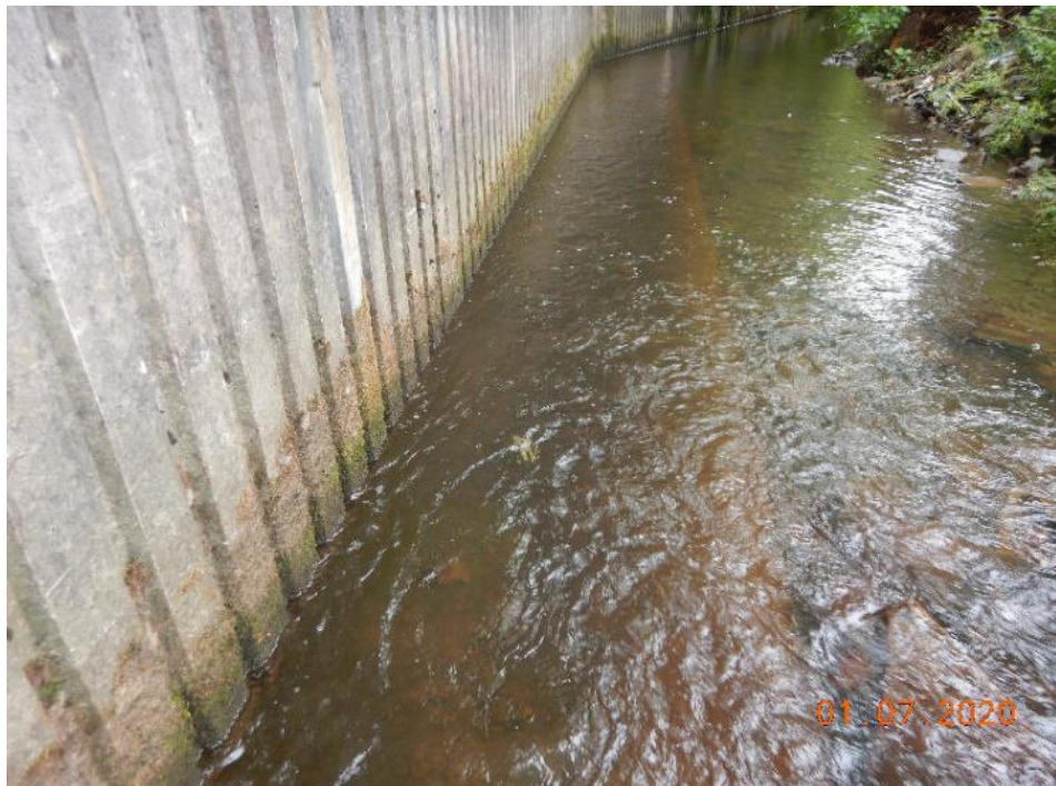
Photo 50 – Concrete apron to the base of the retaining wall (208.8m)
