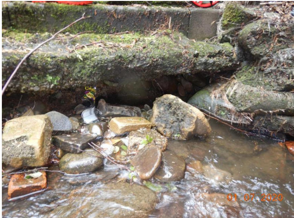
Photo 33 – Undercutting to the concrete toe (145.4m – 156m)
