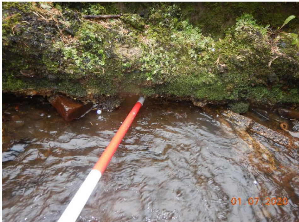
Photo 32 – Scour to the concrete toe (145.4m – 156m)
