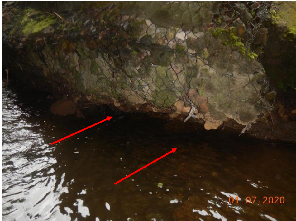
Photo 41 – Undercutting to the gabion basket training wall (163.4m)
