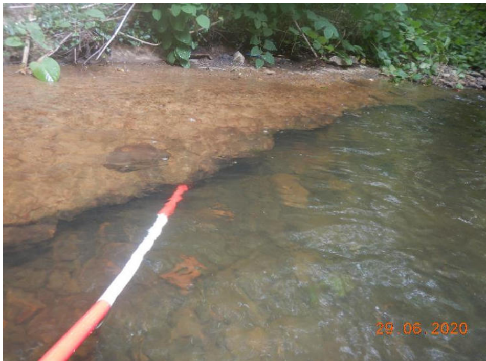
Photo 22 – Undercutting to the right side of the invert (93.3m – 99.7m)
