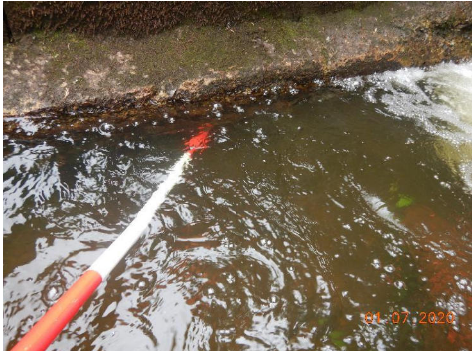
Photo 77 – Undercut to concrete toe (139.7m – 158.8m)
