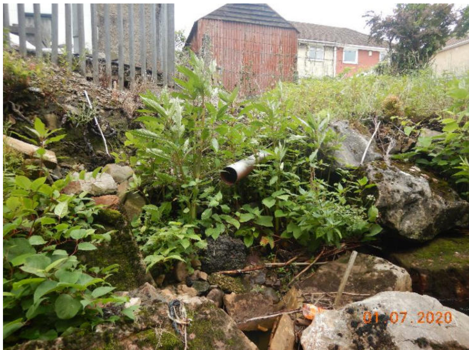
Photo 88 – Displaced rock armour exposing a plastic drainage pipe (275.8m)
