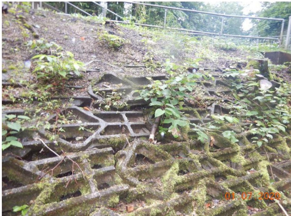
Photo 34 – Displaced concrete (149.9m – 156.6m)
