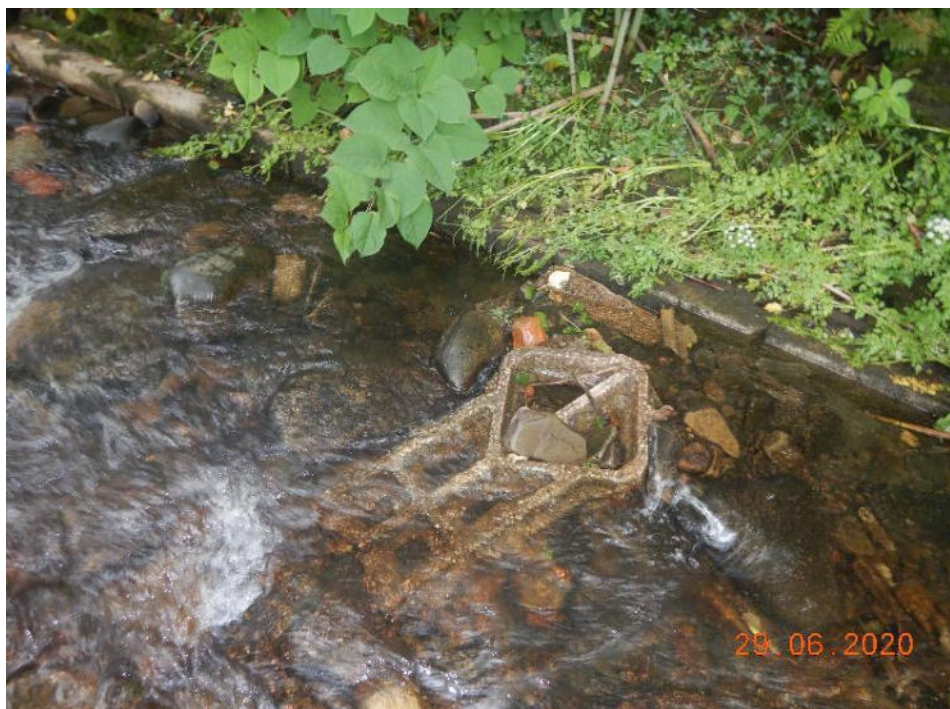
Photo 4 – Sections of the revetment present in the watercourse (0m – 101.2m)
