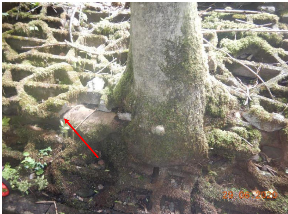
Photo 8 – Tree growth causing displacement of concrete (17.2m)
