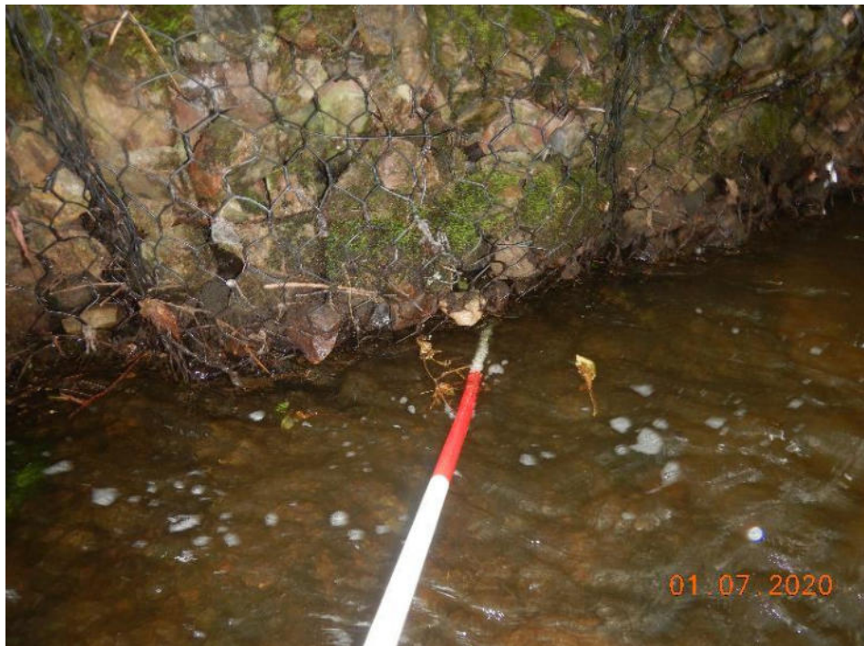
Photo 47 – Undercutting to gabion baskets (185.7m – 192.7m)
