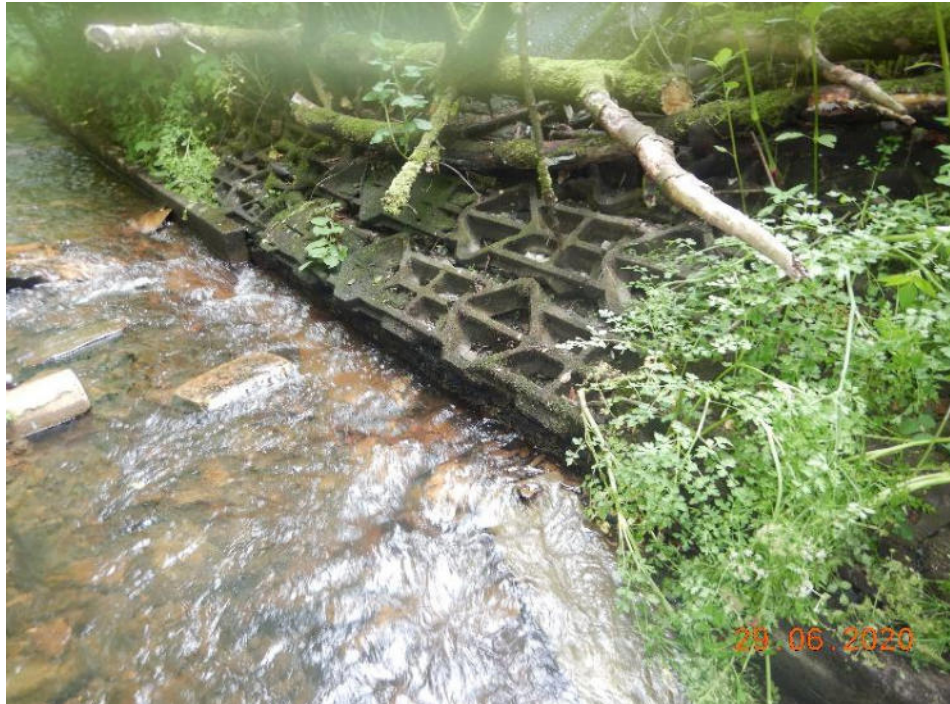
Photo 5 – Missing concrete toe directly upstream of the inspection start point
