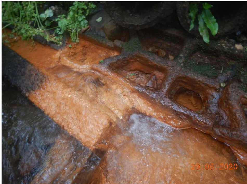
Photo 15 – Water flow through the base of the wall (55m)
