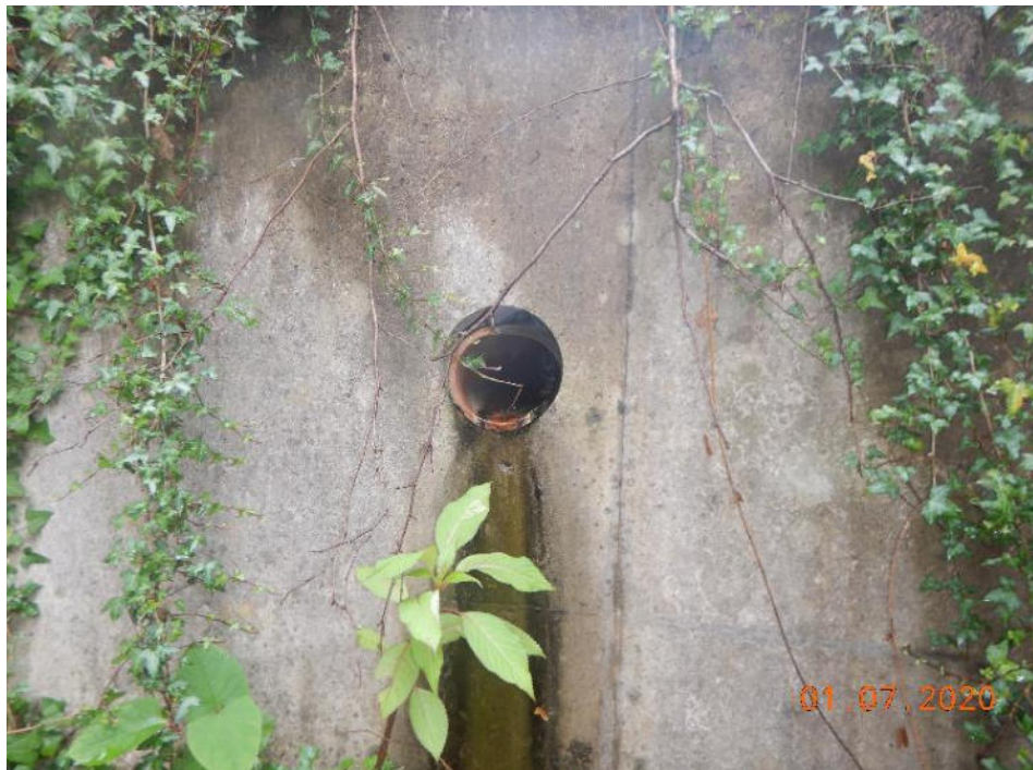
Photo 64 – Clay drainage pipe (409m)
