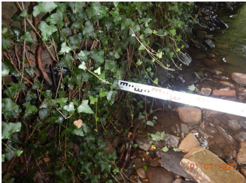
Photo 86 – Scour to the embankment (196m – 203.5m)
