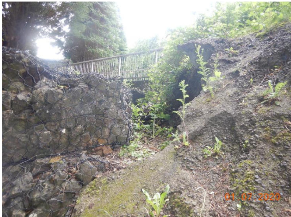
Photo 42 – Void behind the gabion basket training wall (165.4m)
