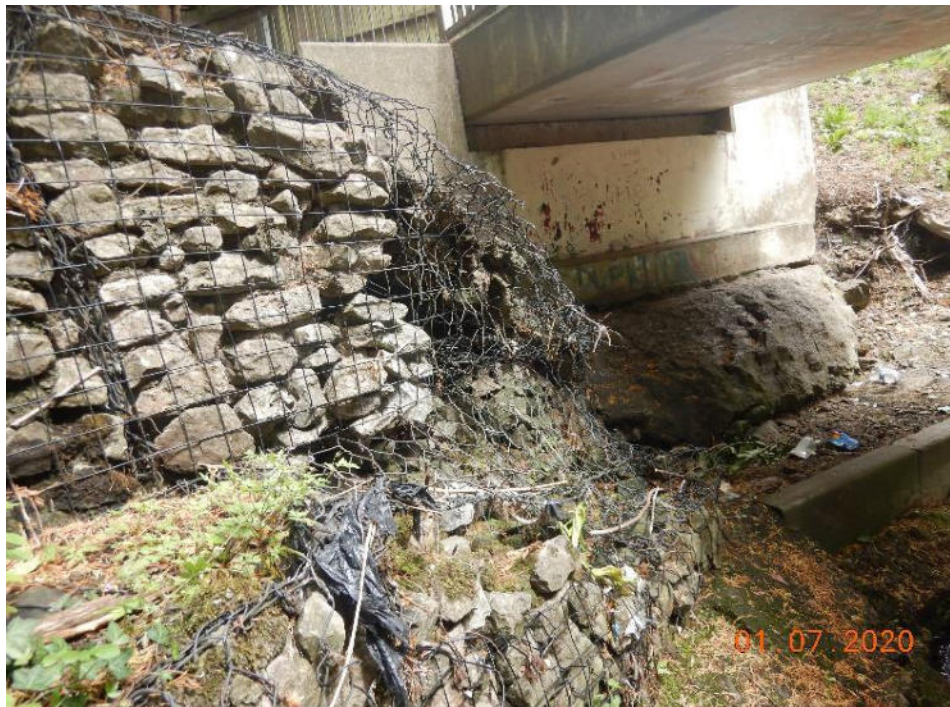
Photo 80 – Failed gabion baskets (159m)
