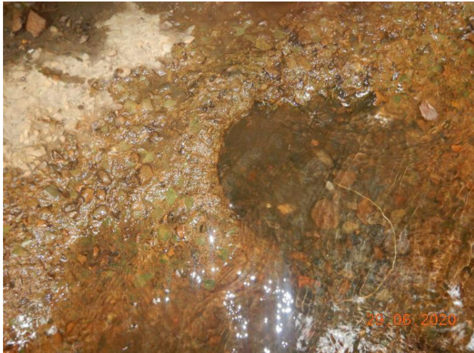
Photo 71 – Scour hole to the right side of the invert (92.9m)
