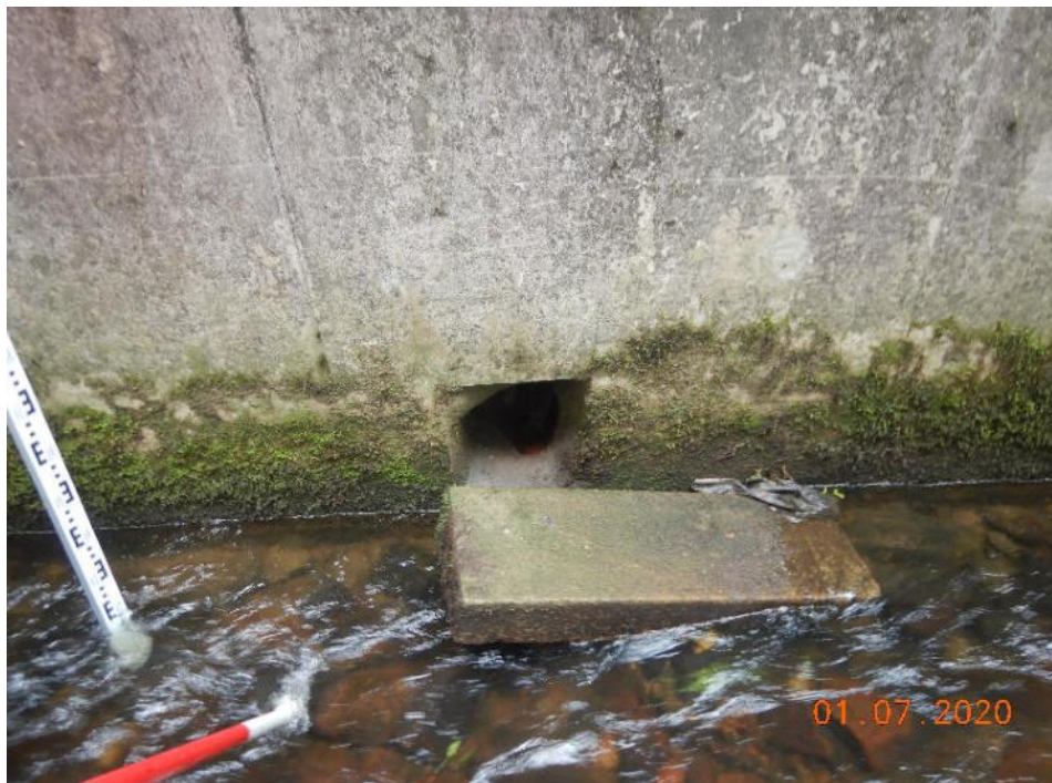
Photo 98 – Clay drainage pipe (364.4m)
