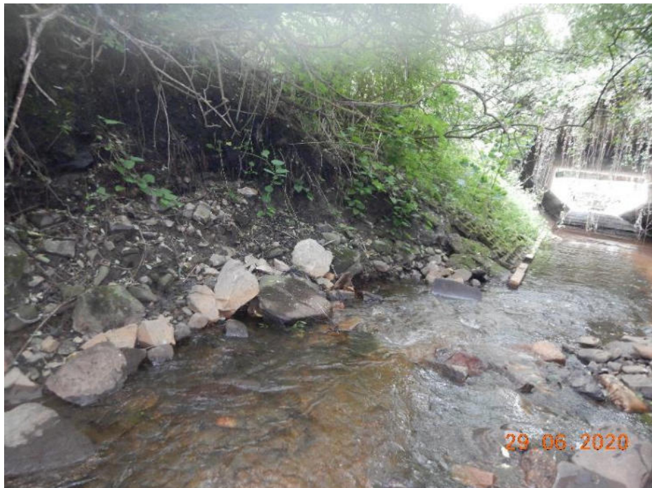
Photo 19 – Failed revetment resulting in scour to the embankment (80.5m – 93.3m)
