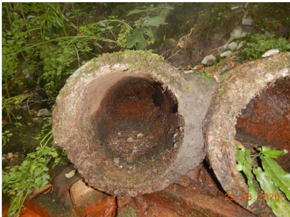
Photo 14 – Fully blocked concrete pipe (55m)
