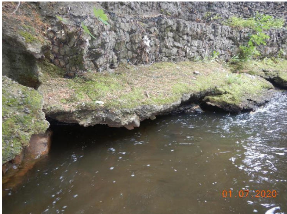
Photo 81 – Undercut to mass concrete supporting gabion baskets (159m – 167m)
