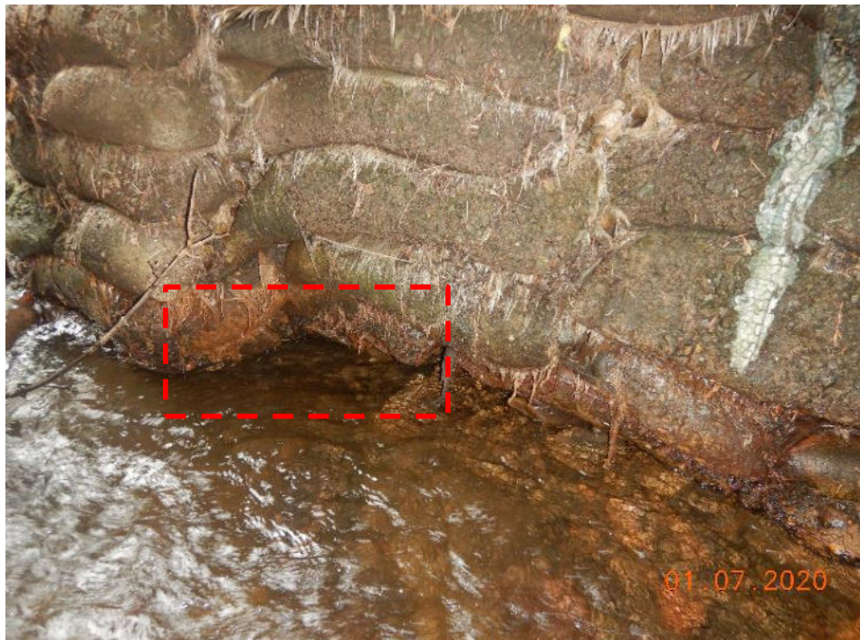
Photo 38 – Scour to concrete bagwork (157m)
