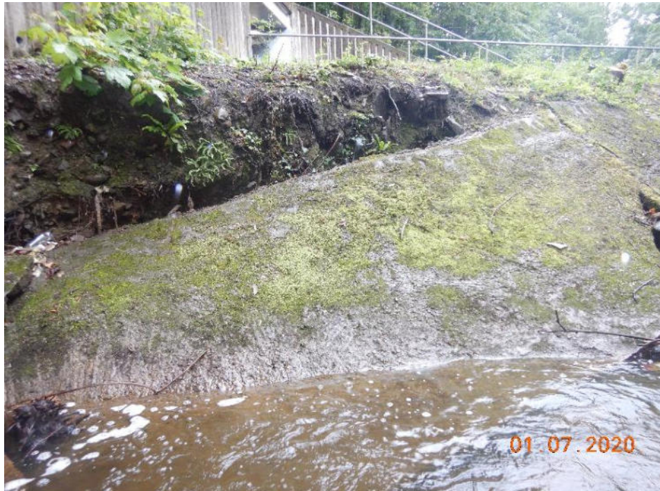
Photo 31 – Failed revetment (139.7m – 145.4m)
