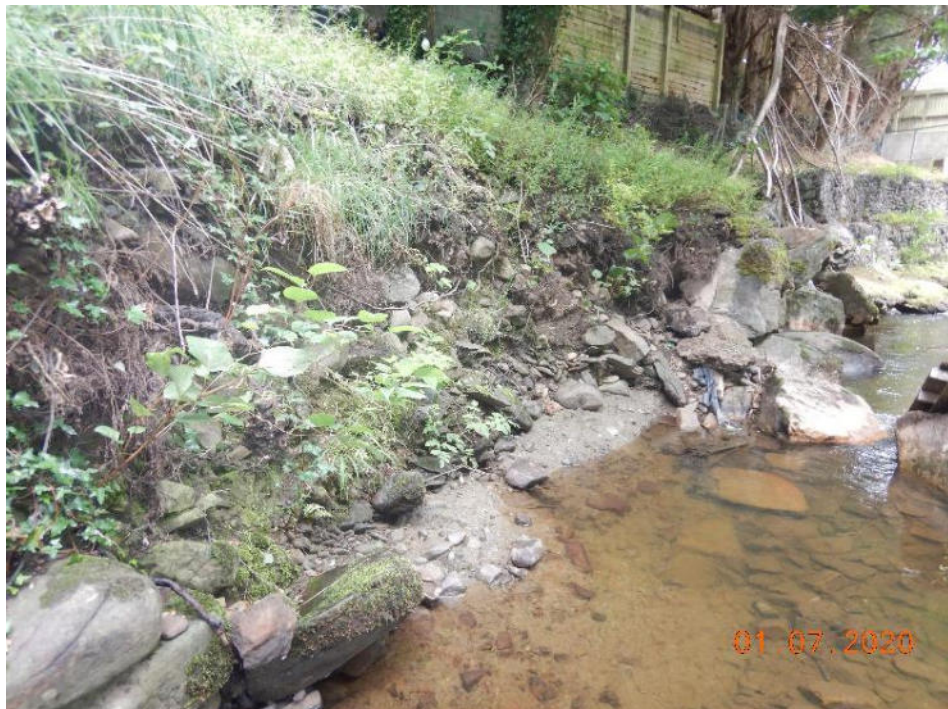
Photo 83 – Scour caused by displaced rock armour (174m – 180m)
