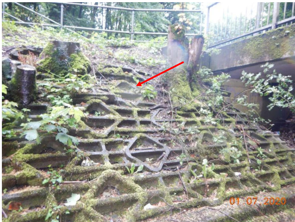
Photo 35 – Displaced concrete and tree stumps (149.9m – 156m)
