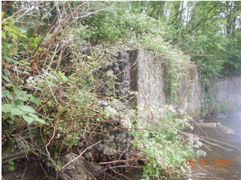
Photo 57 – Dense vegetation growth to gabion baskets (320.5m)
