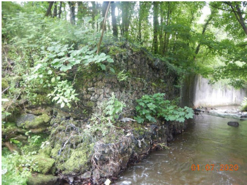
Photo 45 – General view of the gabion basket retaining wall (185.7m – 192.7m)
