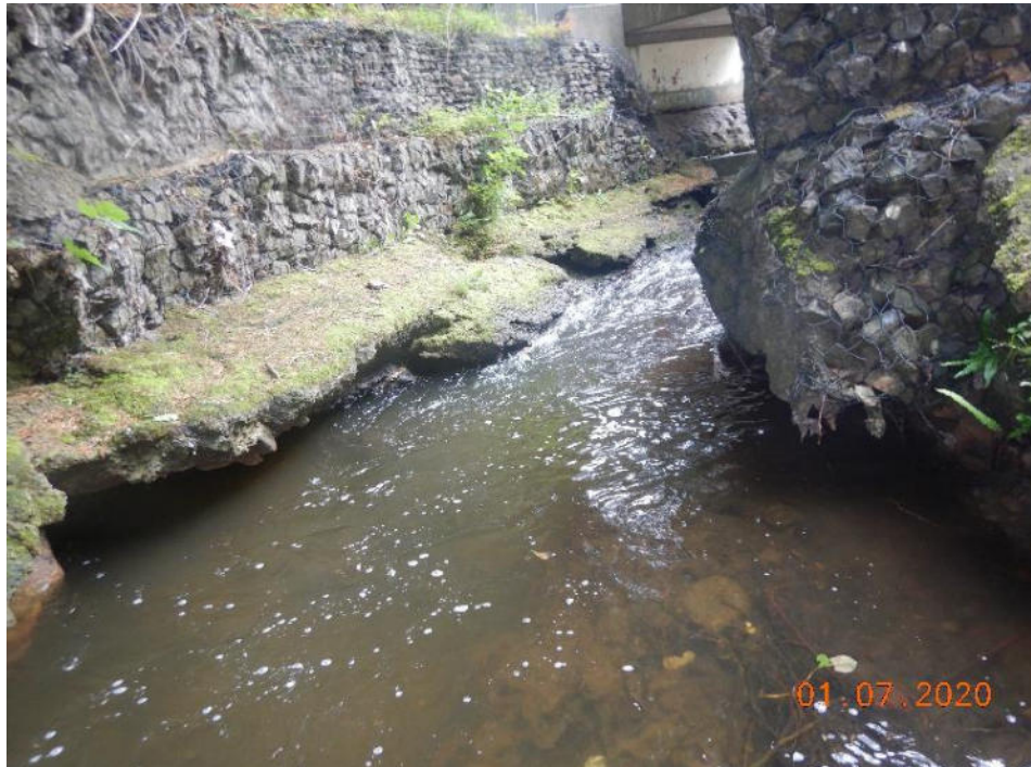
Photo 43 – Remnants of a concrete invert downstream of the footbridge
