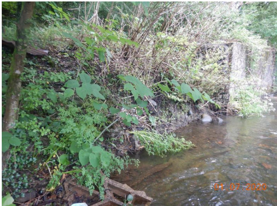
Photo 56 – Failed revetment resulting in scour to the embankment (313.1m – 320.5m)
