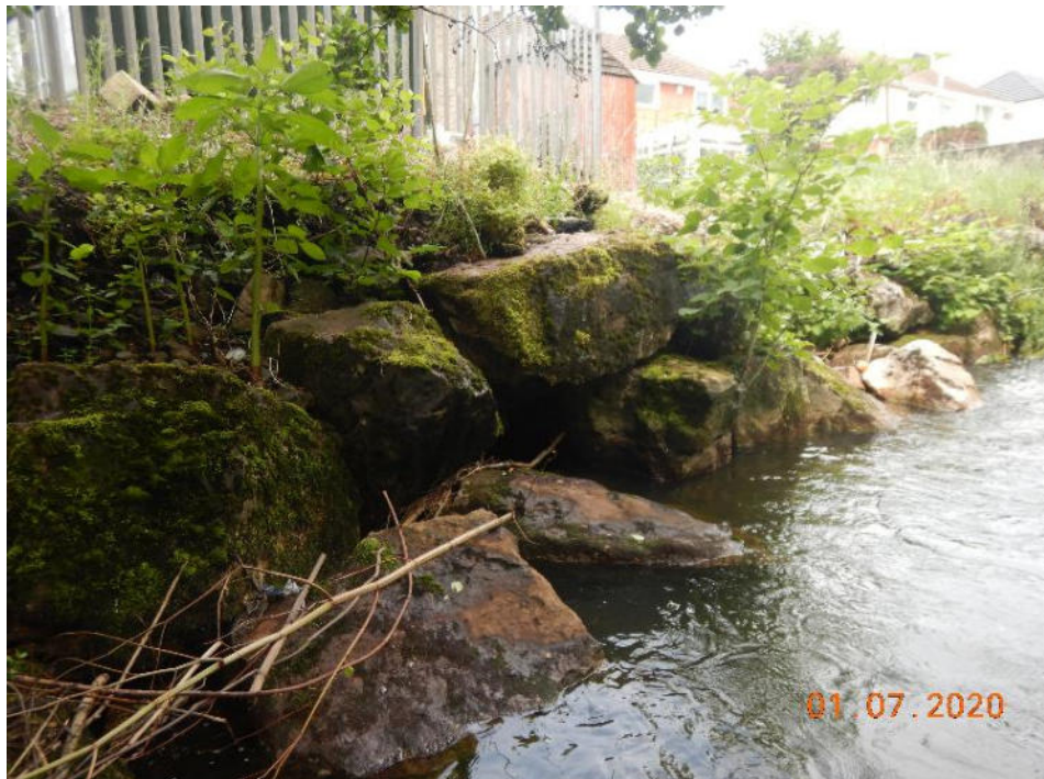
Photo 89 – Displaced rock armour (283m)
