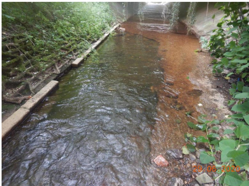
Photo 20 – Missing concrete invert (93.3m – 99.7m)
