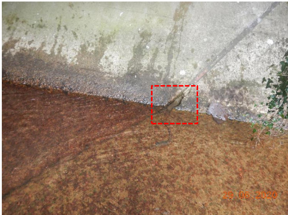
Photo 72 – Missing jointing (101.2m)
