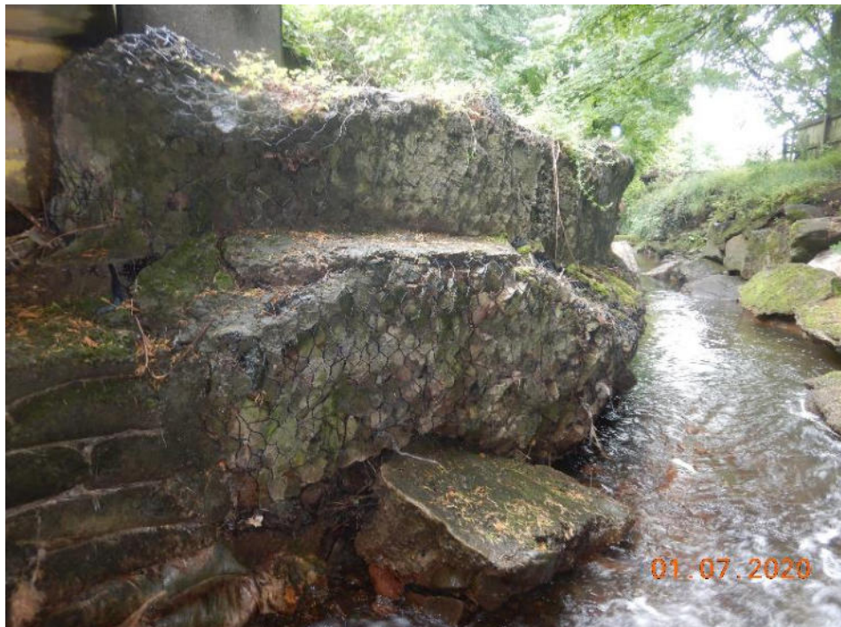
Photo 40 – Condition of the gabion basket training wall (158.8m – 165.4m)
