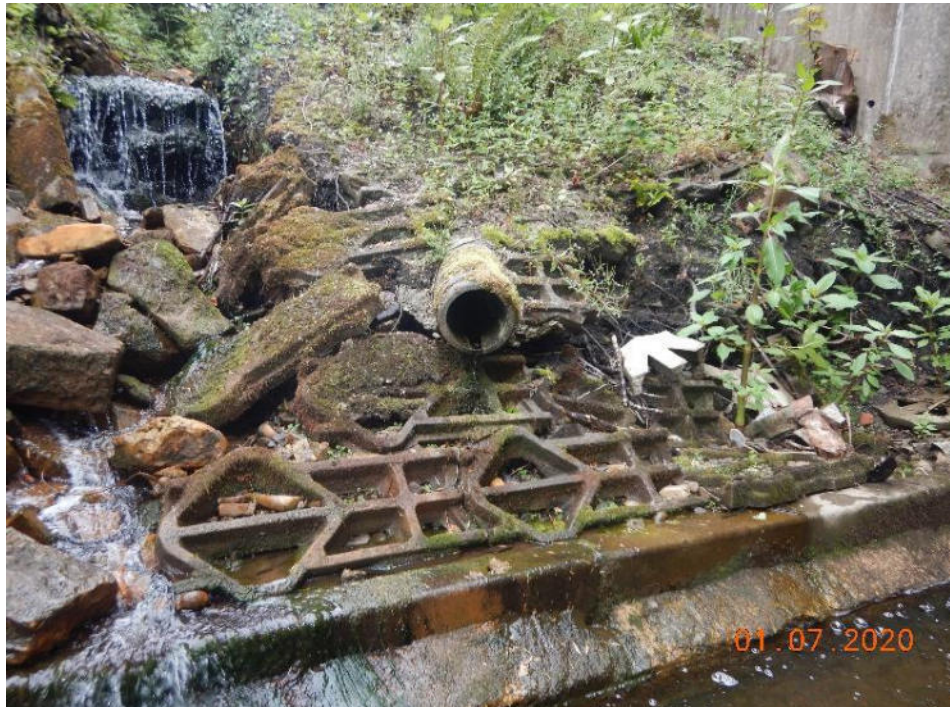
Photo 75 – Missing and displaced concrete surrounding a drainage pipe (144m – 147m)
