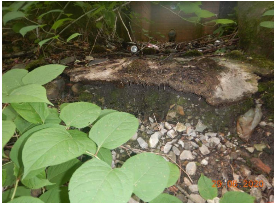
Photo 17 – Undercut to concrete apron (72.6m)
