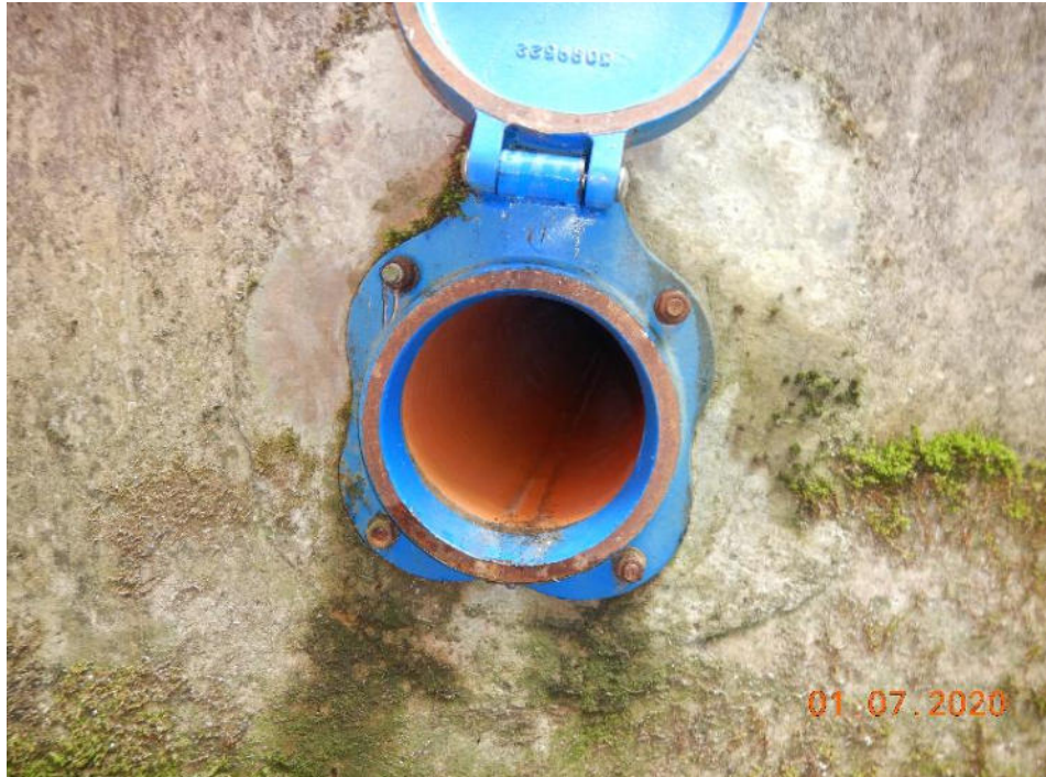
Photo 99 – Clay drainage pipe (368.3m)
