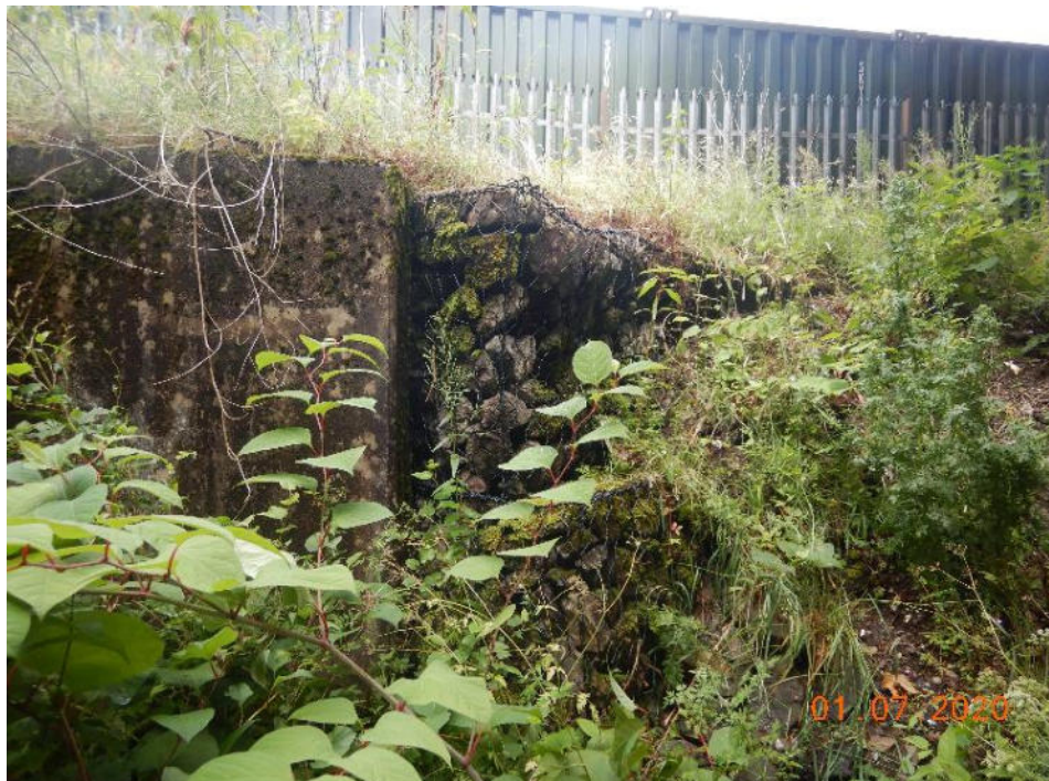
Photo 94 – Condition of gabion baskets (320.5m)
