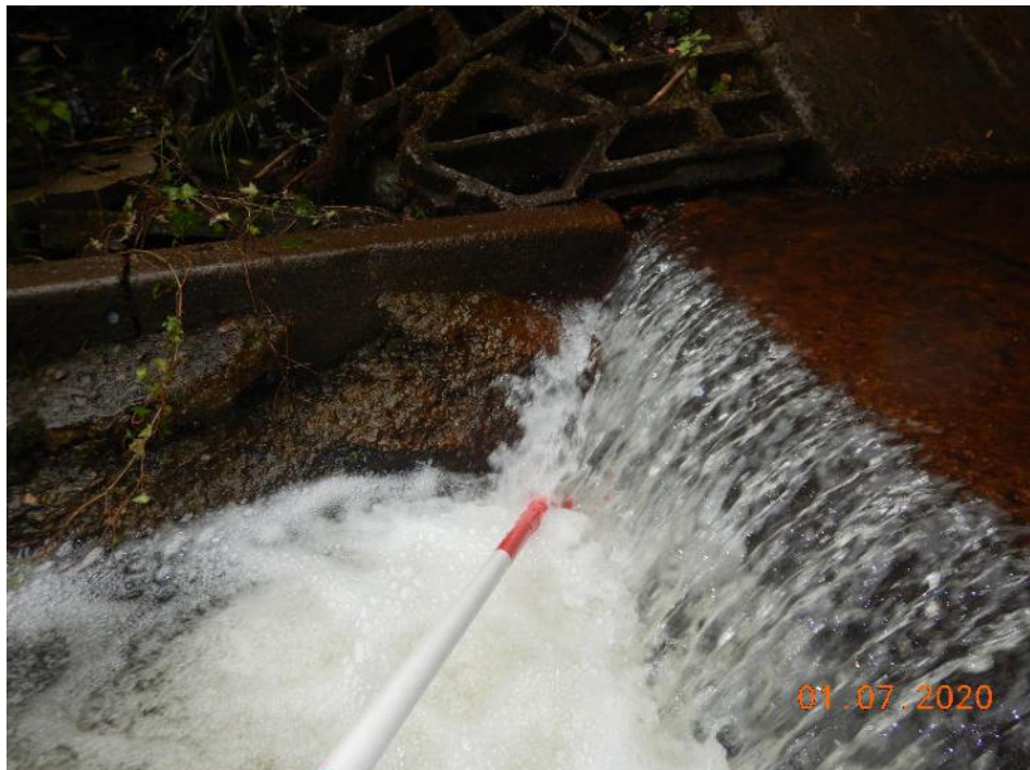
Photo 73 – Location of scour to the weir (139.7m)
