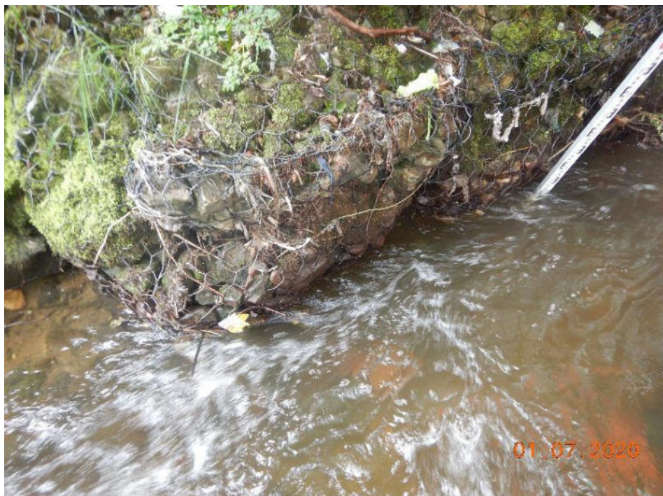
Photo 46 – Bulging and leaning baskets (185.7m – 192.7m)
