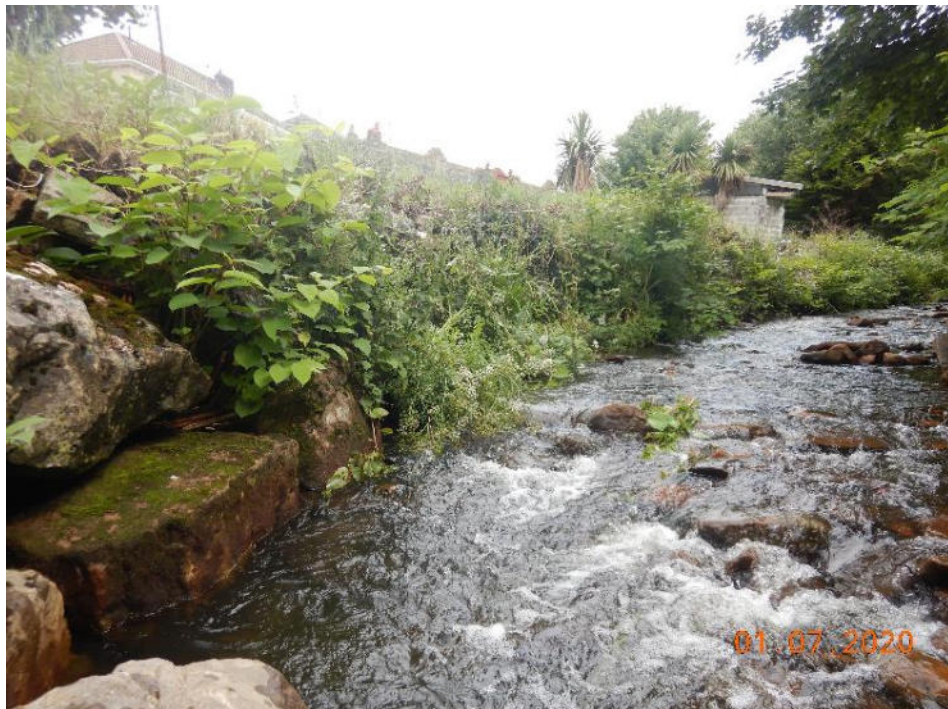
Photo 87 – Dense vegetation growth to rock armour (246.6m – 280m)
