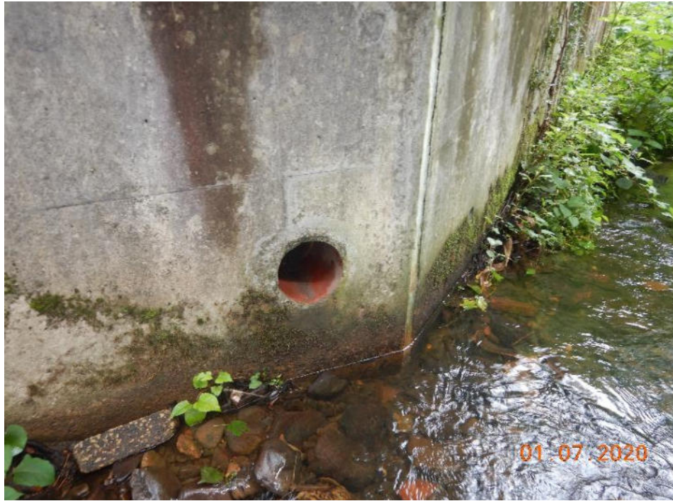
Photo 97 – Clay drainage pipe (332.1m)
