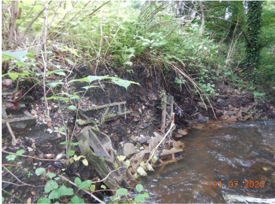
Photo 53 – Failed revetment (296.1m – 306.4m)
