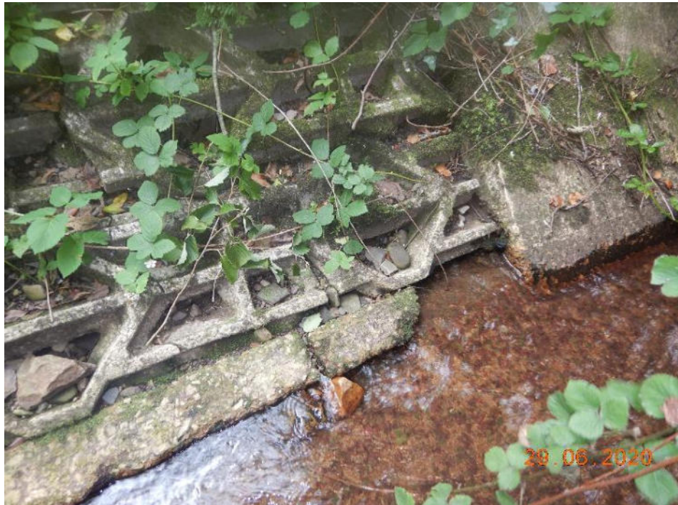
Photo 23 – Missing concrete toe (100.6m)
