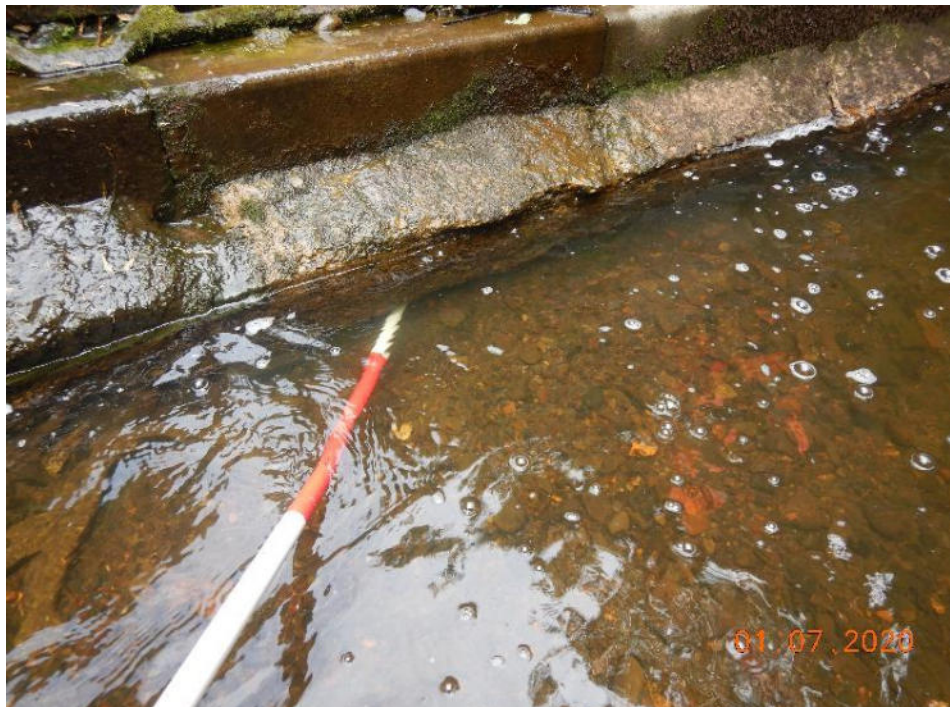
Photo 76 – Undercut to concrete toe (139.7m – 158.8m)
