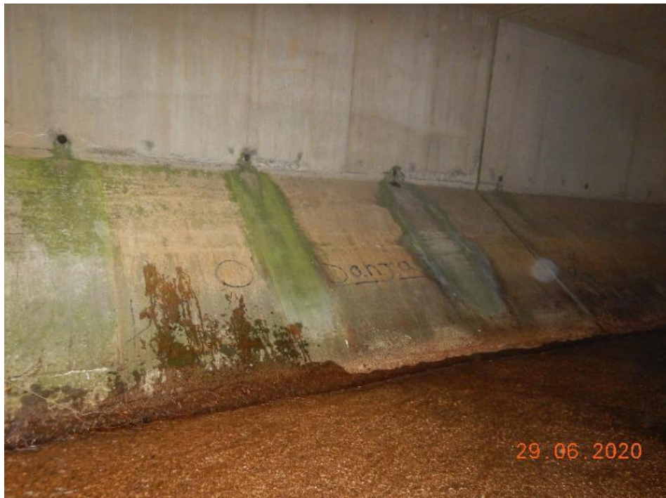
Photo 25 – White and green coloured infiltration (101.2m – 139.7m)
