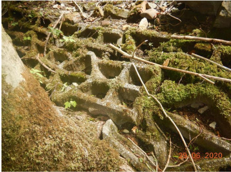
Photo 9 – Tree growth causing displacement of concrete (19.3m)
