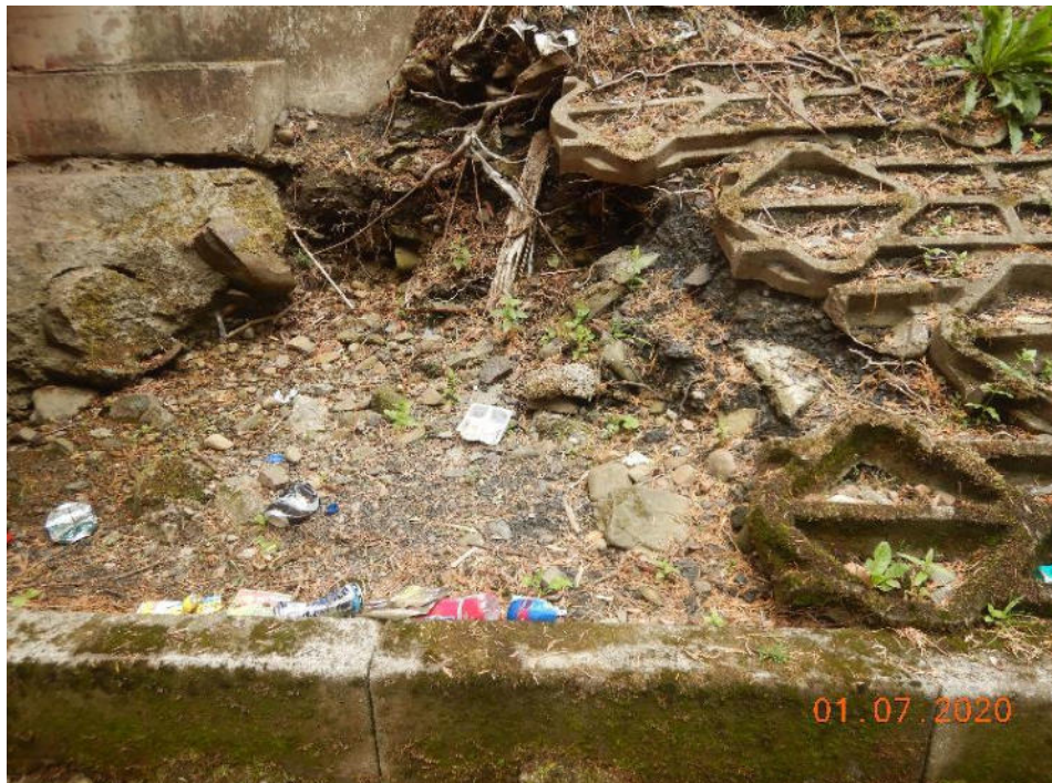
Photo 78 – Failed revetment (154m – 156m)
