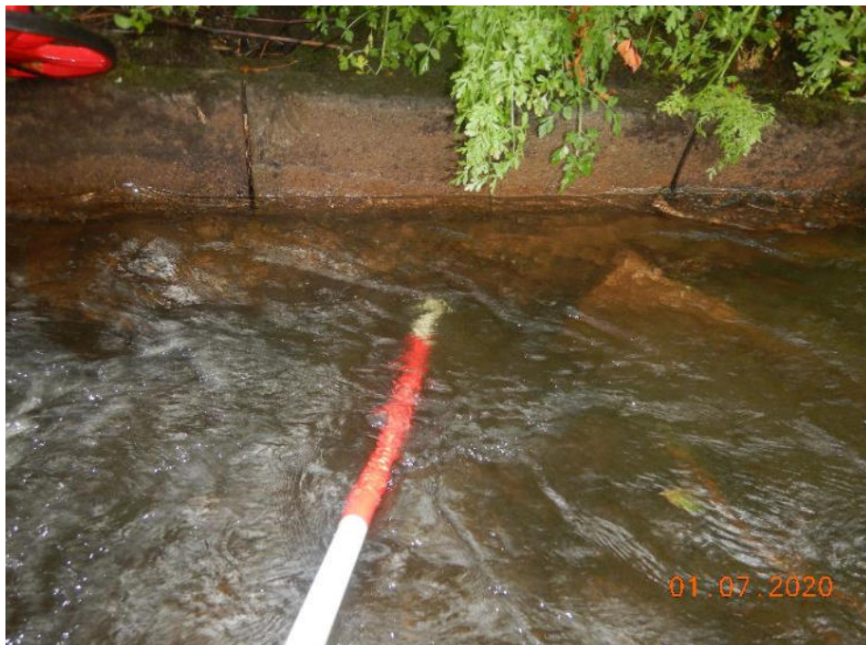
Photo 54 – Undercut to concrete toe (307.7m – 313.1m)
