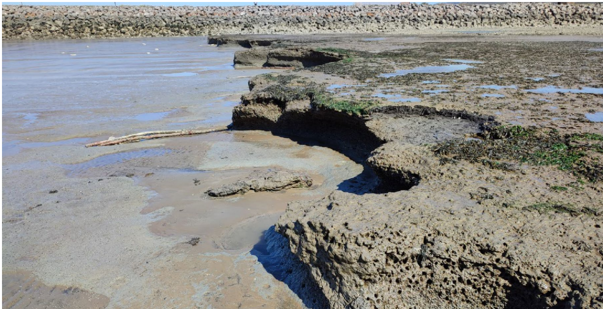
Image 3. Eroding peat edge (right) and exposed clay (left)
