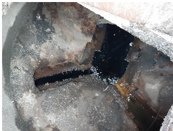
Figure 1: Sample point/ inspection chamber
