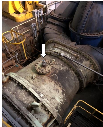
Pump and Suction Pressure Transducer
