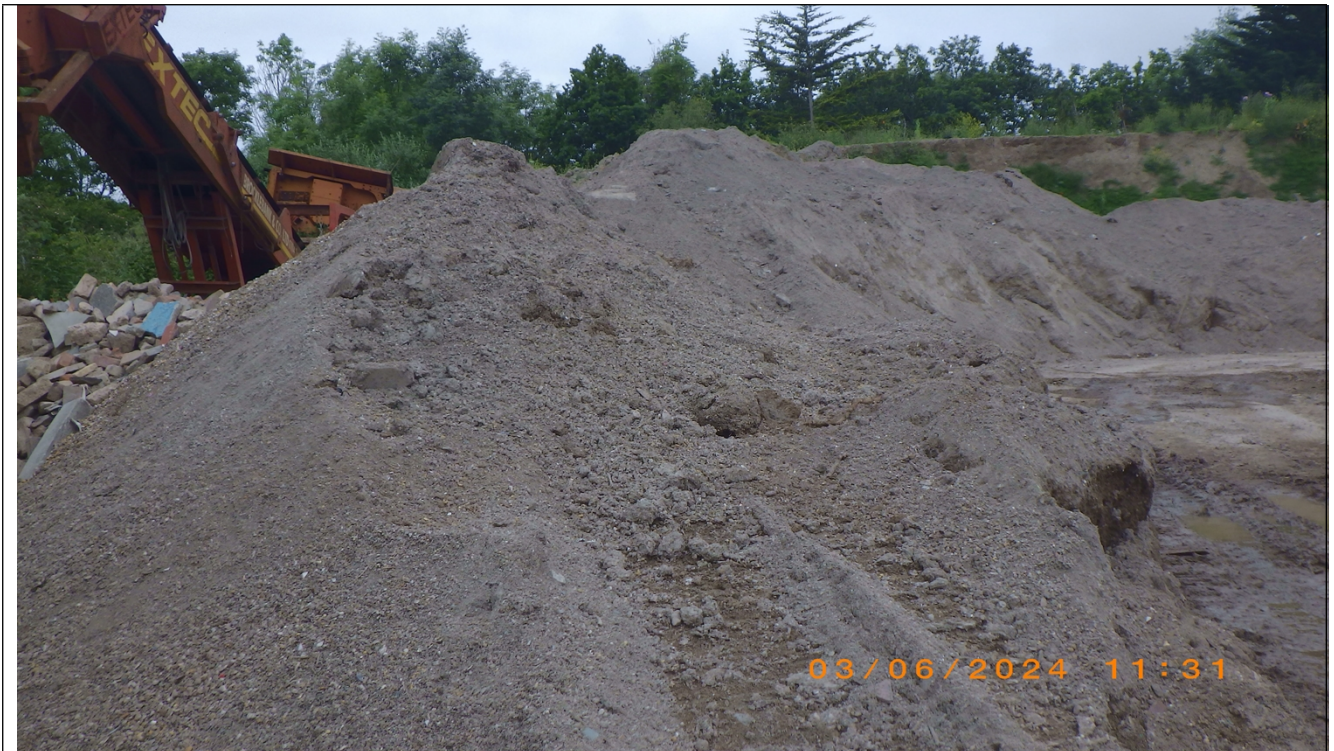
Photograph showing stockpile of waste fines
