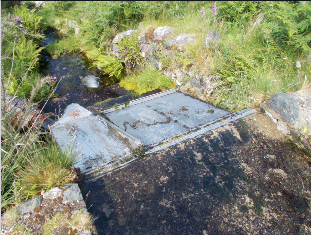
Image 3 shows the compensation plate used for the seasonal flow variations
