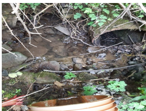
Figure 2: Tributary flowing clearly at discharge point 4
