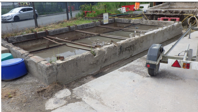
Figure 6: Site visit photo – Settlement tanks on site at the time of the visit working as designed.
