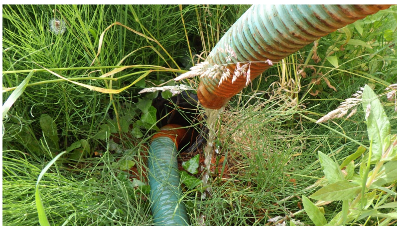
Figure 7: Site visit photo – The discharge of pumped mine water observed during the visit.
