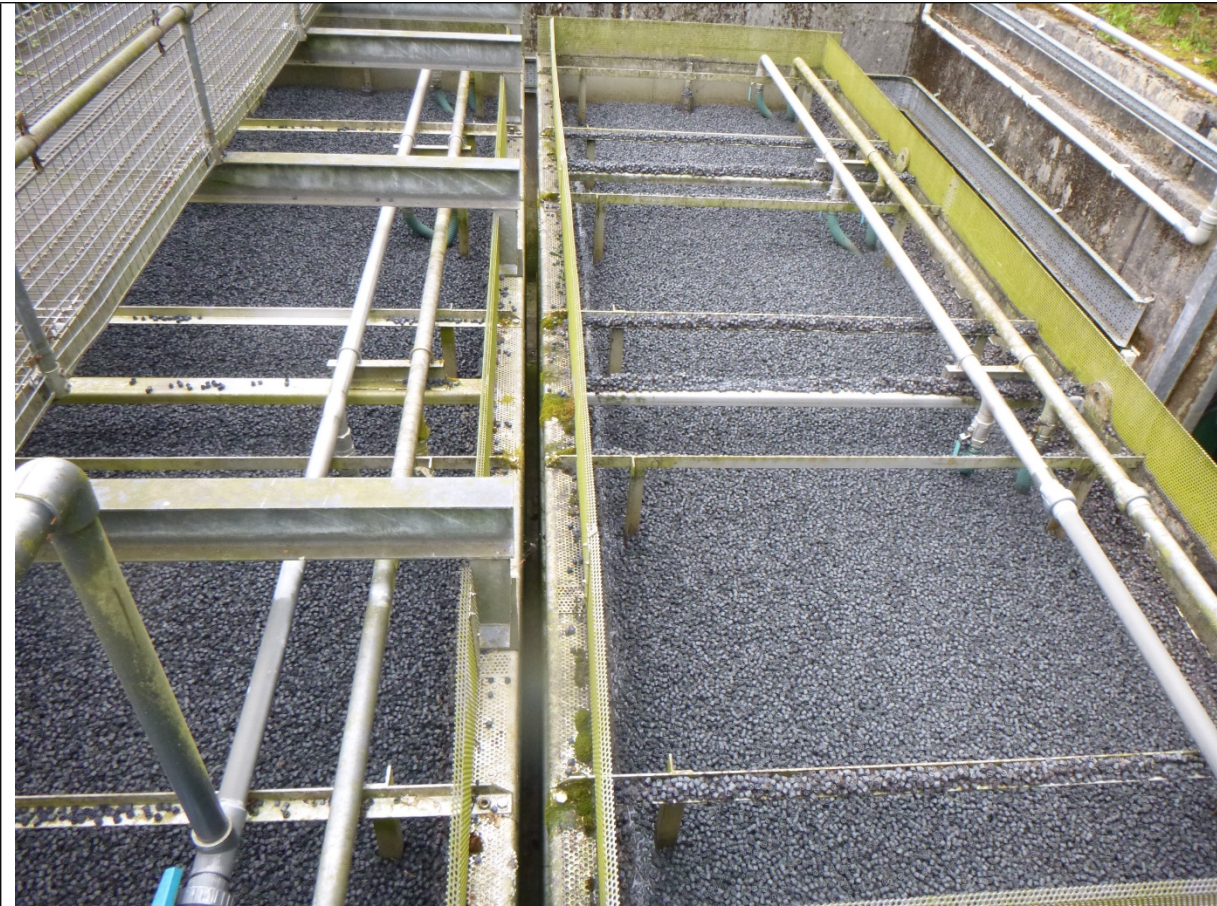
Figure 1 Filter beds at works made up of plastic media
