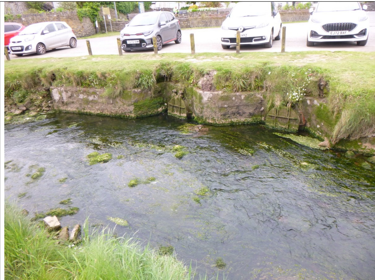
Figure 2. Flap valves where the SPS Emergency overflow is, no evidence of fungus, or odour present in the watercourse.
