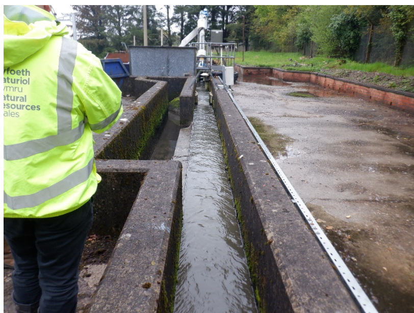
Figure 1. Flows entering works, the screw screen can be seen in the centre of the photo.
