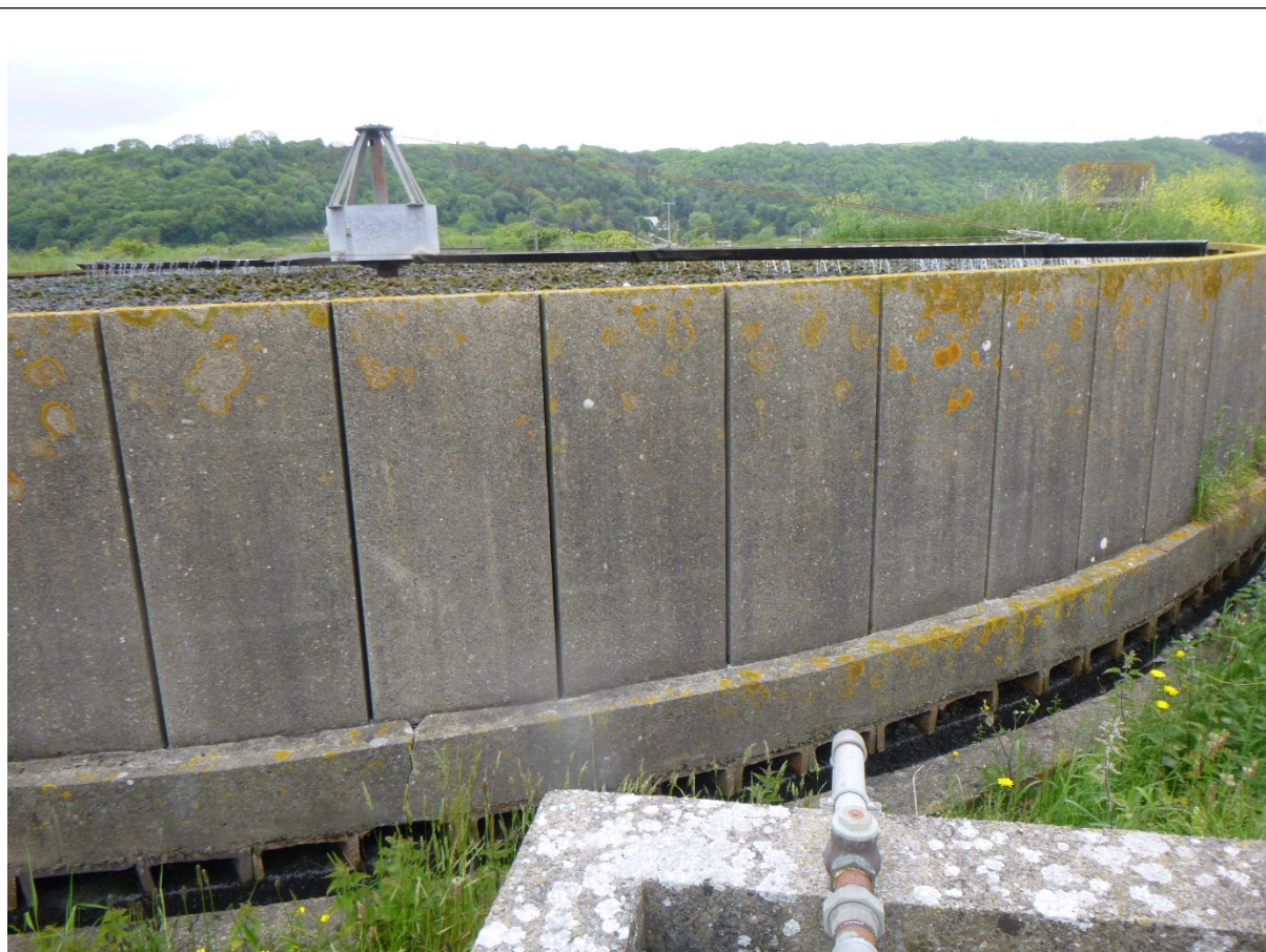
Filter bed, no concern of growth with the arms moving freely and unhindered.
