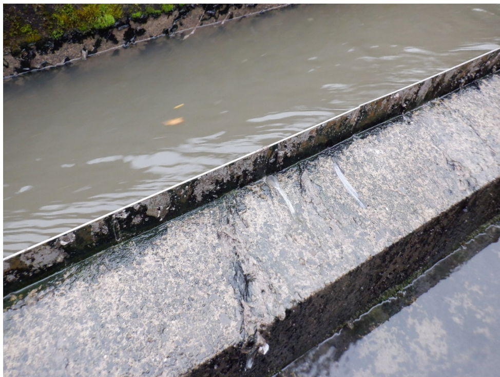
Figure 2. Leak in weir, discharging sewage when flows are below the height of the weir.
