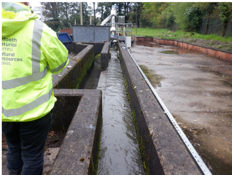
Figure 1 Location of the CSO weir with the drum screen located on the left side channel.
