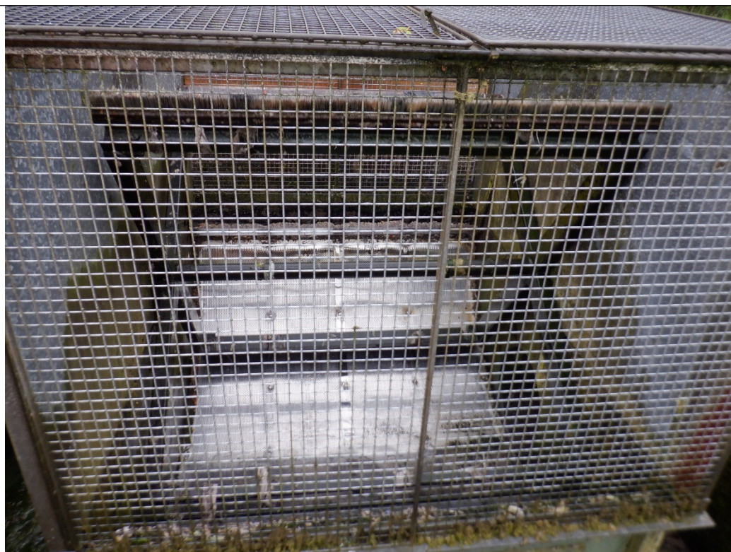
Figure 3 Drum screen on the CSO channel before it is spilled to the environment.
