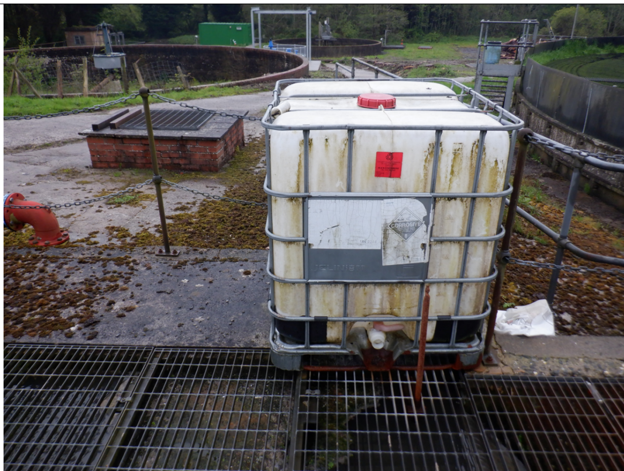
Figure 8 IBC incorrectly stored with no bund present.
