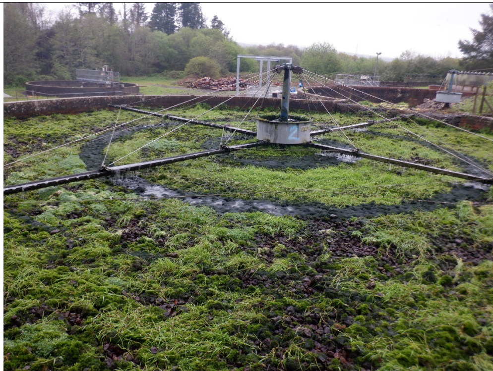
Figure 5 Further treatment of effluent through old filter bed.
