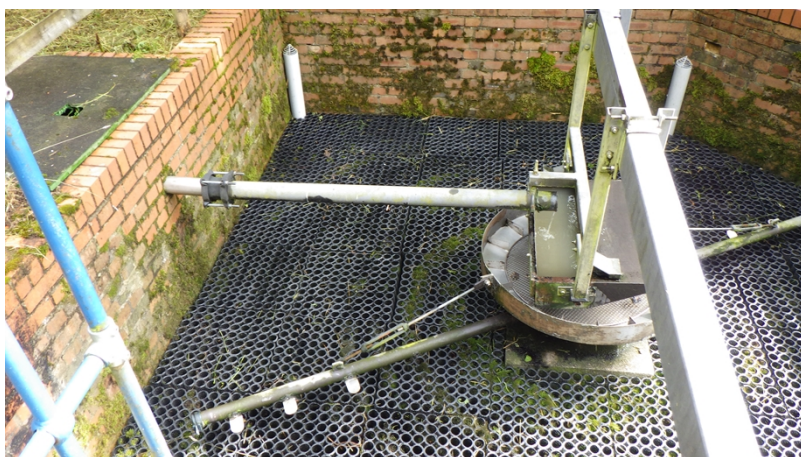
Figure 2 – Site visit photo: Filter bed showing no signs of build up of solids or fungus.
