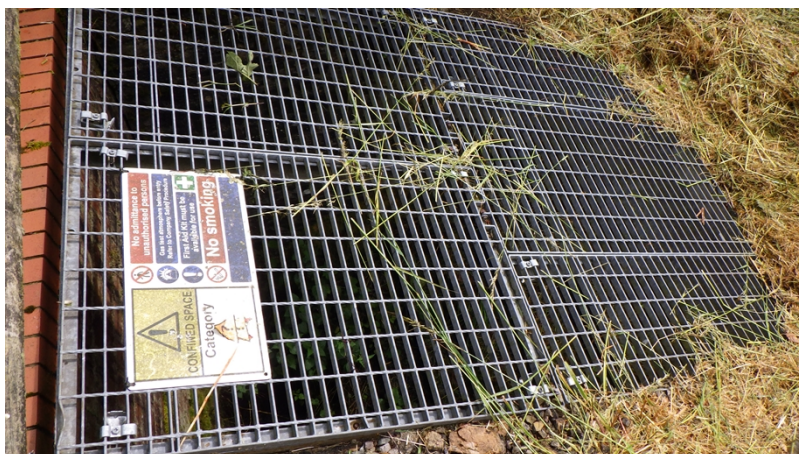
Figure 4 – Site visit photo: Access to soakaway and sample point.
