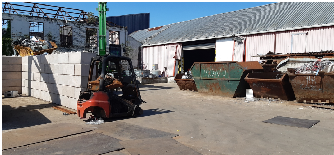
Photo 2 - Impermeable surface in good condition and secondary containment measures (background)
