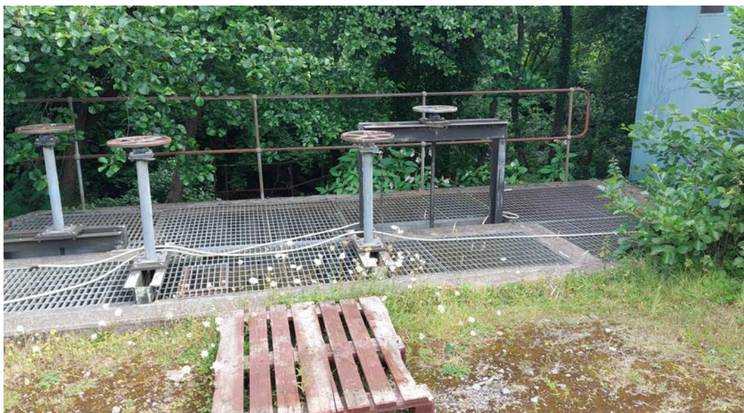
Photograph 10-4: Effluent outfall diversion chamber
