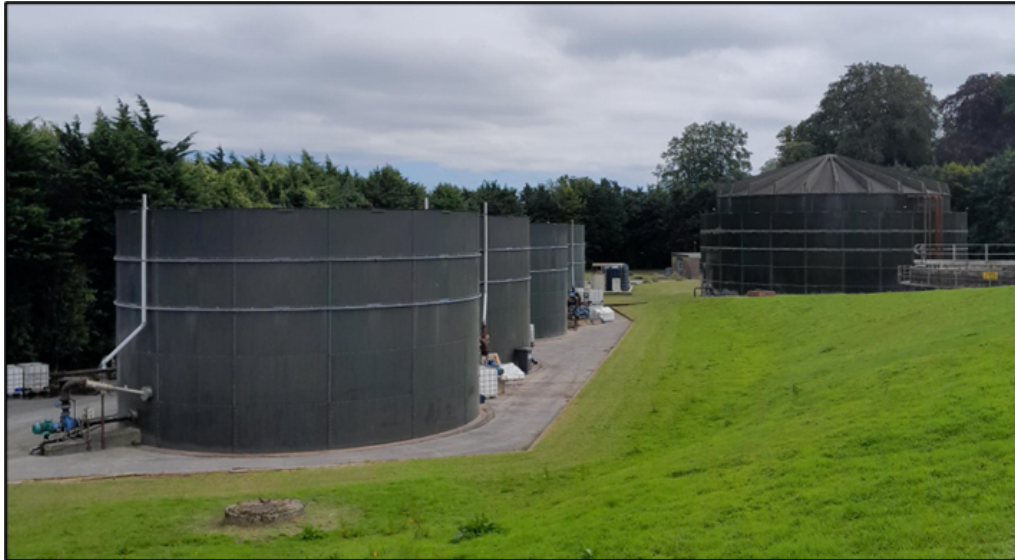
Image 3 – showing tanks 5, 6, 8, and 9 on the left, taken on 19 July 2024
