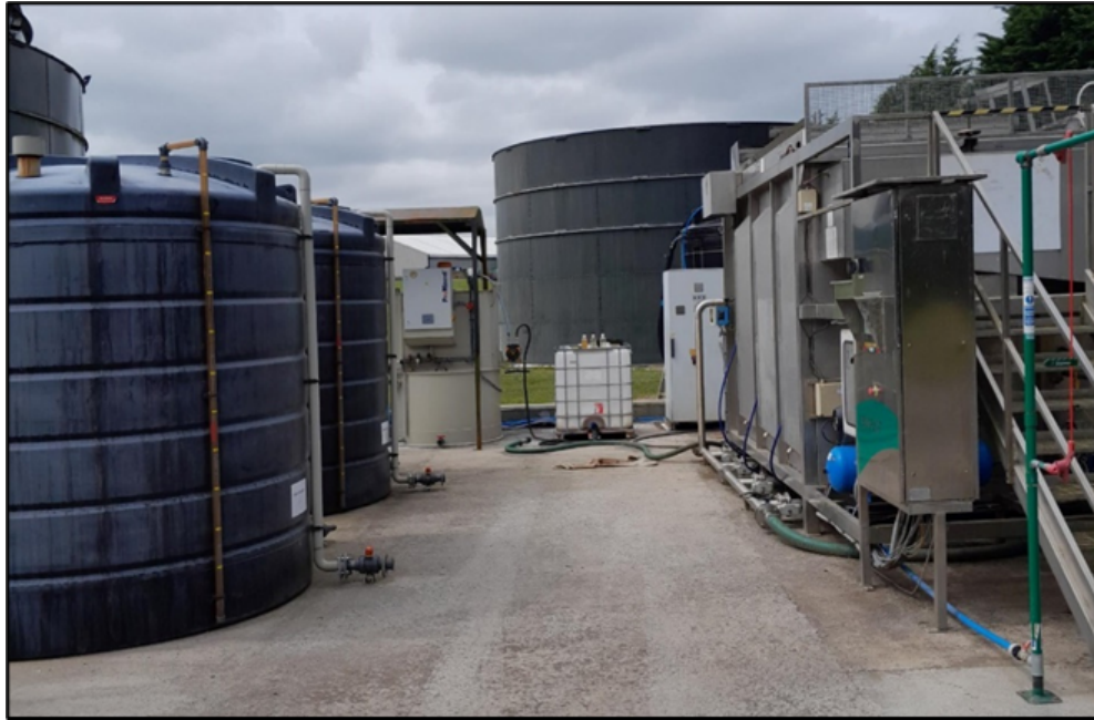
Image 4 – showing the DAF unit and chemical dosing vessels, taken on 19 July 2024
