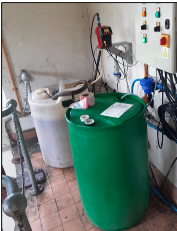
Image 5 – showing the antiffoam dosing system housed in a unit, taken on 19 July 2024
