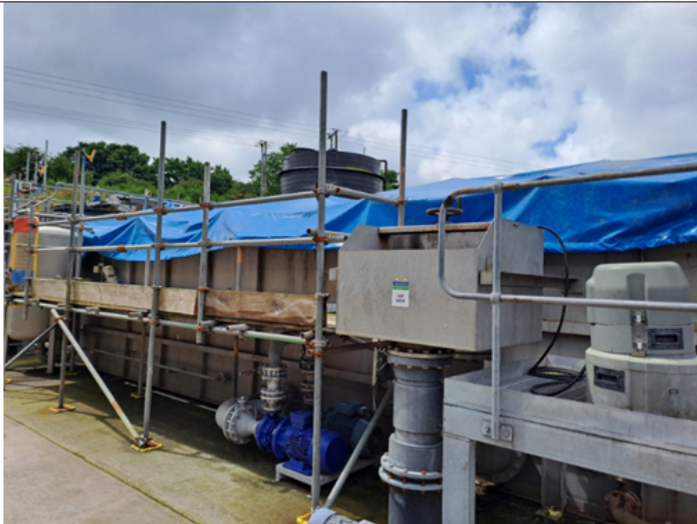
Image 10 – Primary DAF with plastic cover
