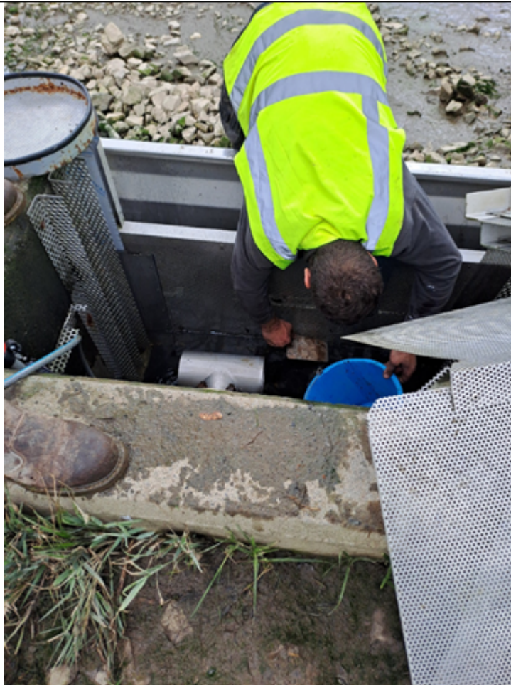
Image 05 – Operators collecting the material accumulated on the screen to be weighed for reporting.
