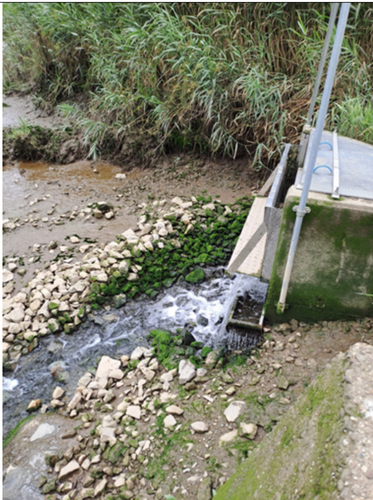
Image 06 – Screen reassembled, and flow returned to normal rate.
