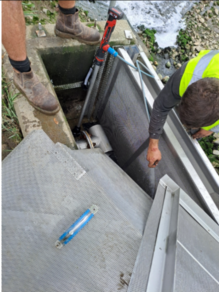
Image 04 – Operators flushing the screen prior to collecting the material.
