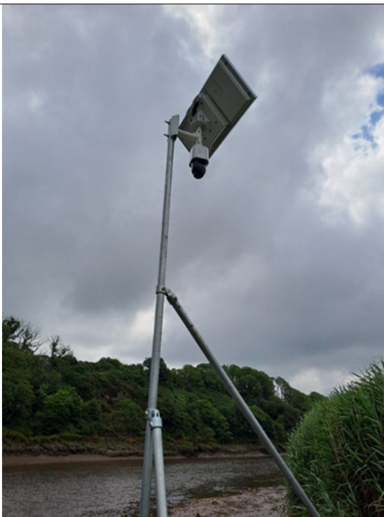
Image 07 – CCTV camera positioned above the First Milk outfall for 24/7 monitoring.
