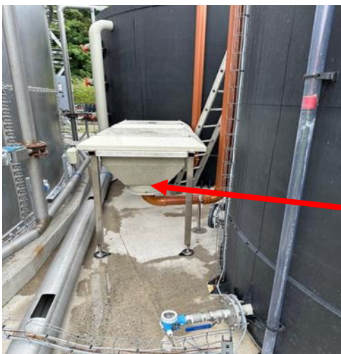
Passive carbon filters used at Dairy Partners
