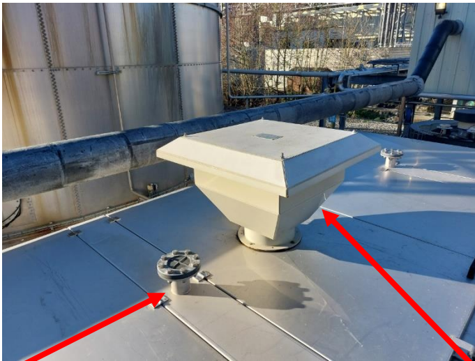
Manufacturer’s aperture for a passive odour filter system
