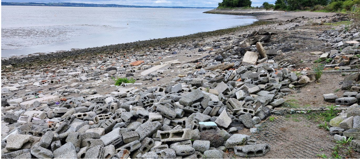
Image 4. View (southeast) of the southeastern part of remedial area
