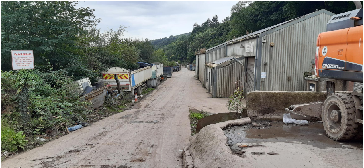
Photo 5 - On site waste transfer activities on the 'bottom yard'
