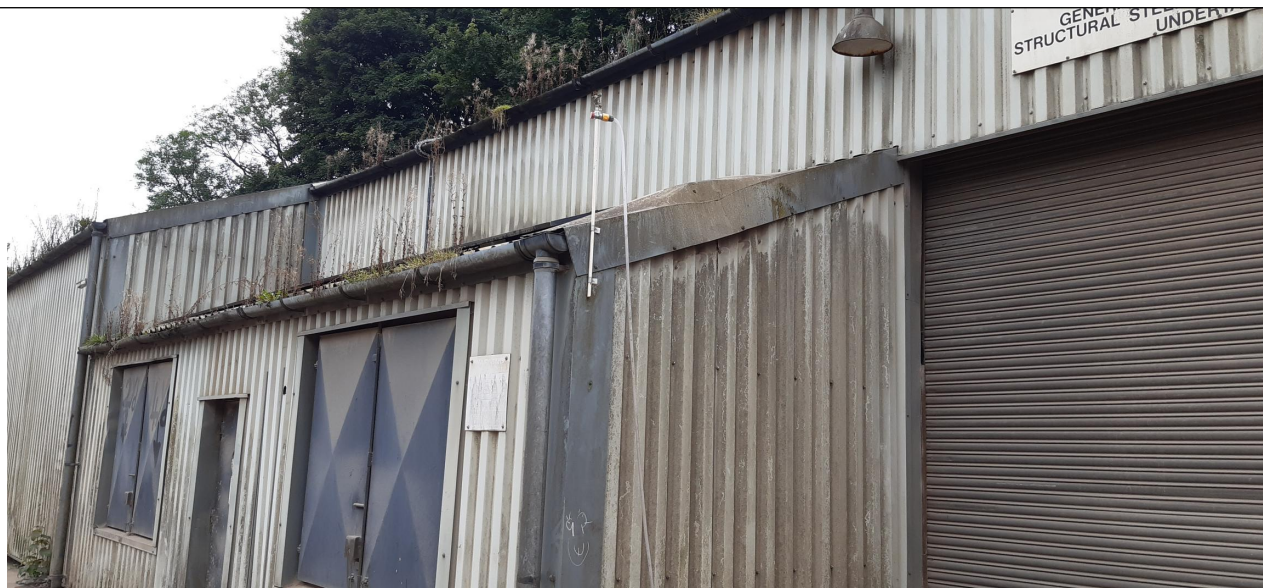
Photo 8 - Sprinkler system (top middle) located at CWS Ltd
