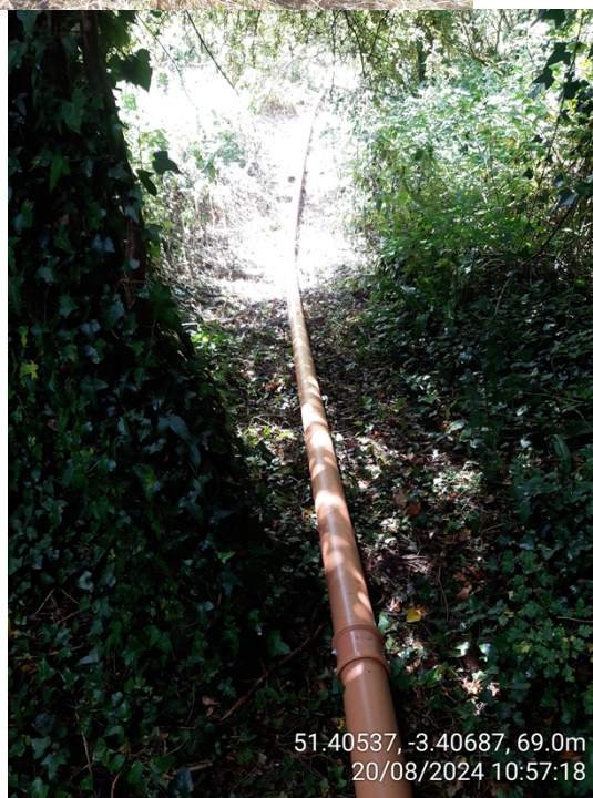
(Left) Newly installed access gate to discharge. (Right) Newly installed pipeline to discharge point.
