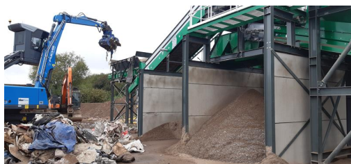
Photo 1, start of picking line loaded by machine.
