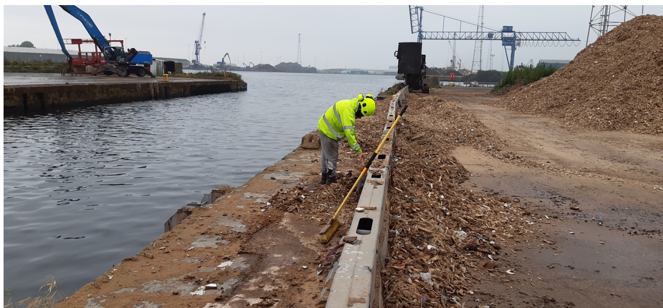
Photo 4 - ABP Site to the left of the blue shipping containers
